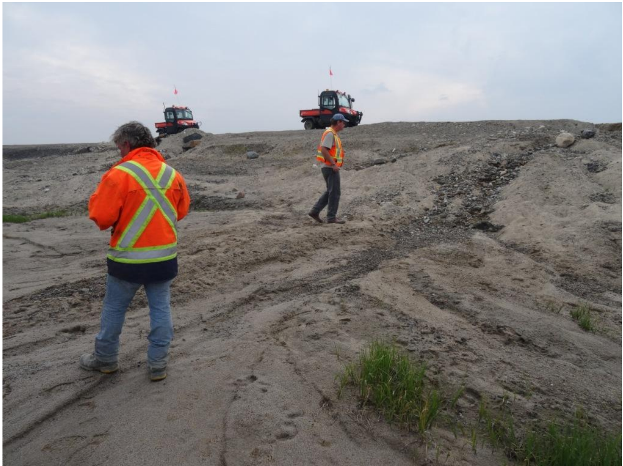
Figure 13. Recurring wash-out location at Dam 6. Aerial view in Figure 17.
