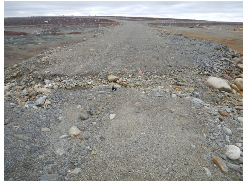
Lupin Dam L erosion channel
