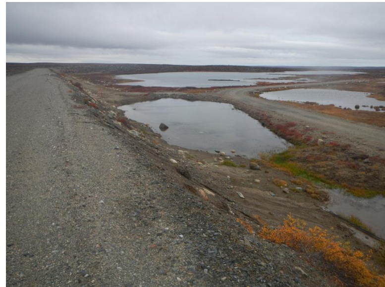
Lupin Dam 2 DS slope and seepage collection pond
