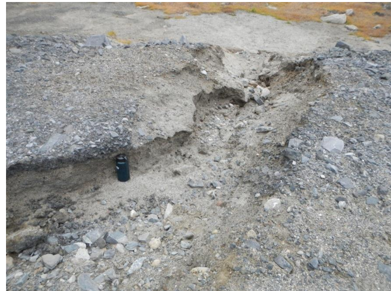
Lupin Dam 4 eastern DS slope erosion
