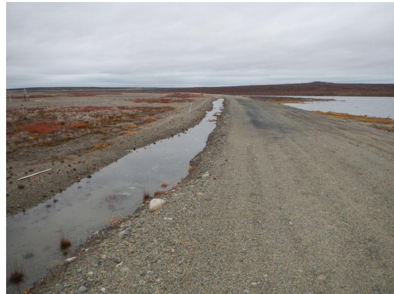
Lupin Dam 3 Crest with ponding in ditch
