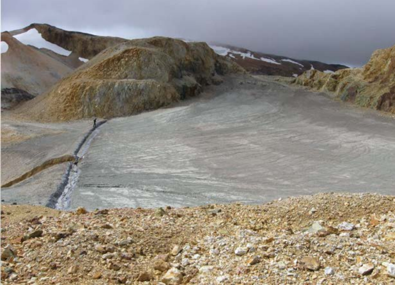
Filling of open pit and profiling to natural environment
