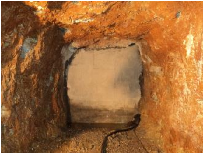
Closure of underground access
