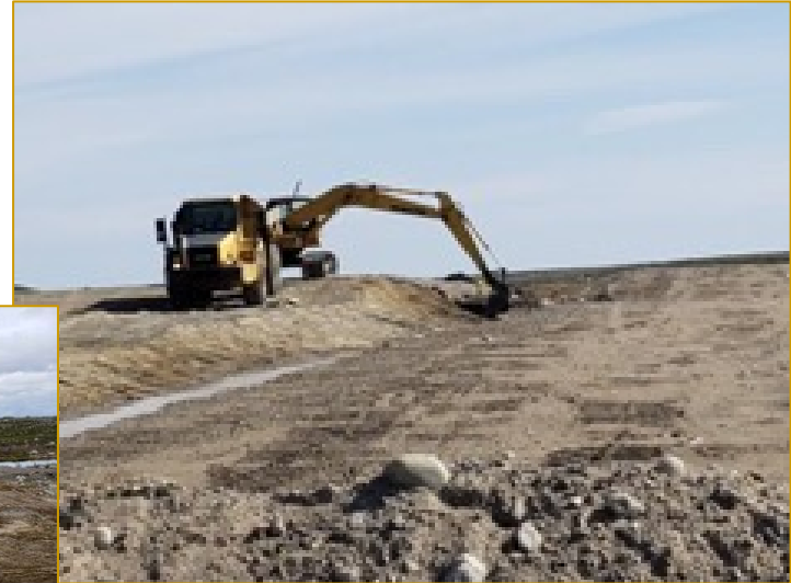
Repairs to KDam Crest (erosion gullies) July 16, 2019
