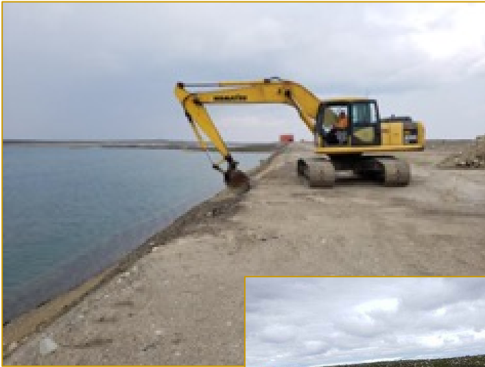
Repairs to KDam Crest (erosion gullies) July 16, 2019
