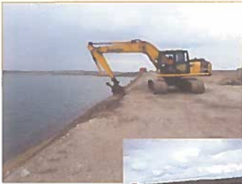
Repairs to KDam Crest (erosion gullies) July 16, 2019
