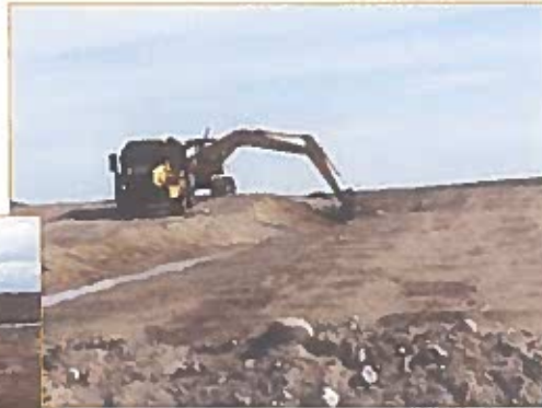
Repairs to KDam Crest (erosion gullies) July 16, 2019
