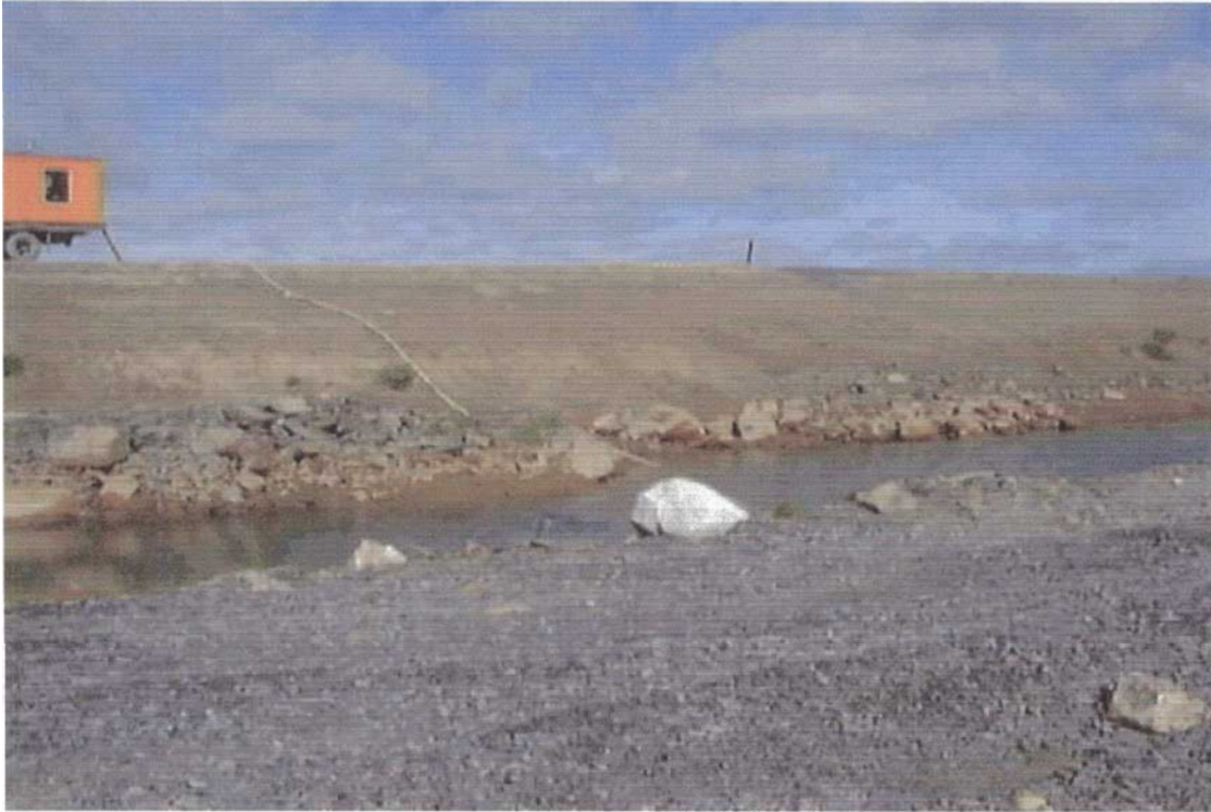
figure 4. Pumping, into Cell 4, of water pooled by Cofferd Dam; 2001/08/11.
