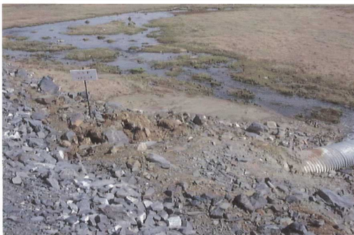
figure 5. Signs of berm erosion along the discharge culvert at SNP 925-14; 2001/07/08.
