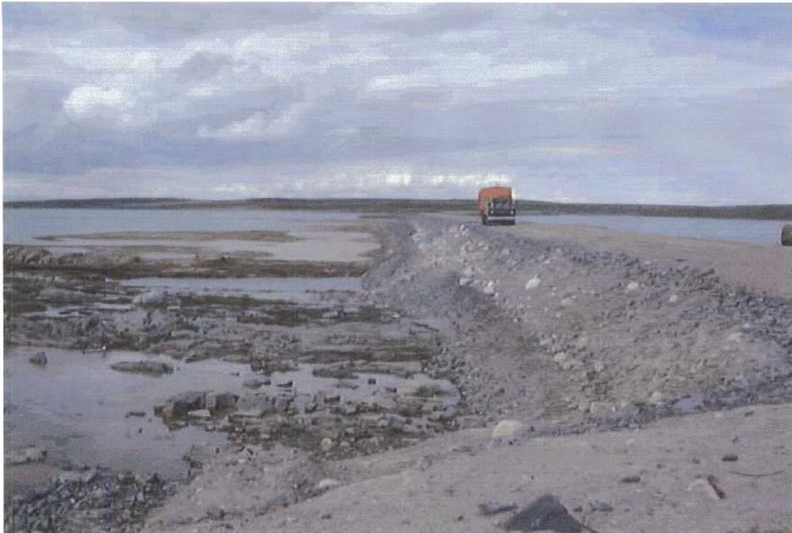
figure 1. Seepage zone along M Dam, separating Cell 5 from Pond 2; 2001/07/08.
