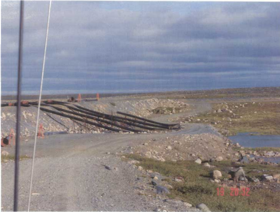
Photo # 13. Tailings Pond 2 Siphon Discharge Structure. Dam 1A location of Tailings discharge SNP-925-10 sample location.
