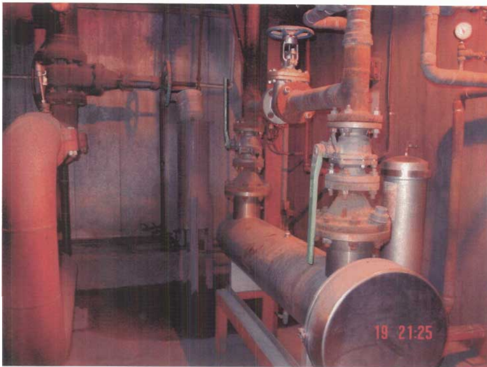
Photo # 3. Ultra Violet Disinfection System for potable water in milling complex.
