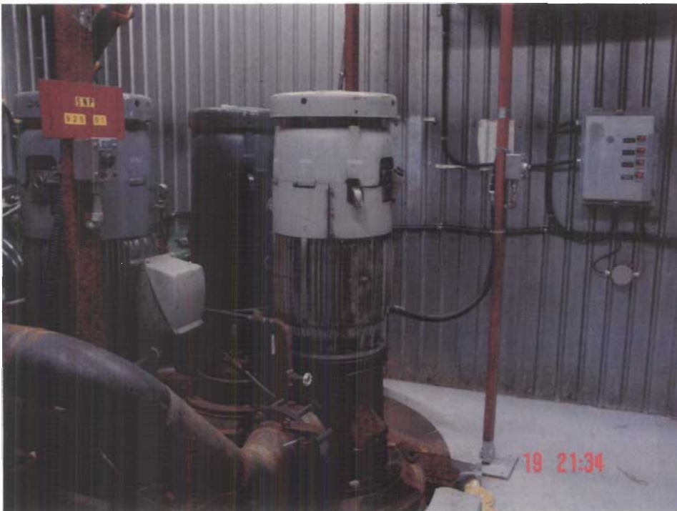
Photo # 2. Some leakage from water supply pump in foreground at Water Intake Facility, SNP station -01.
