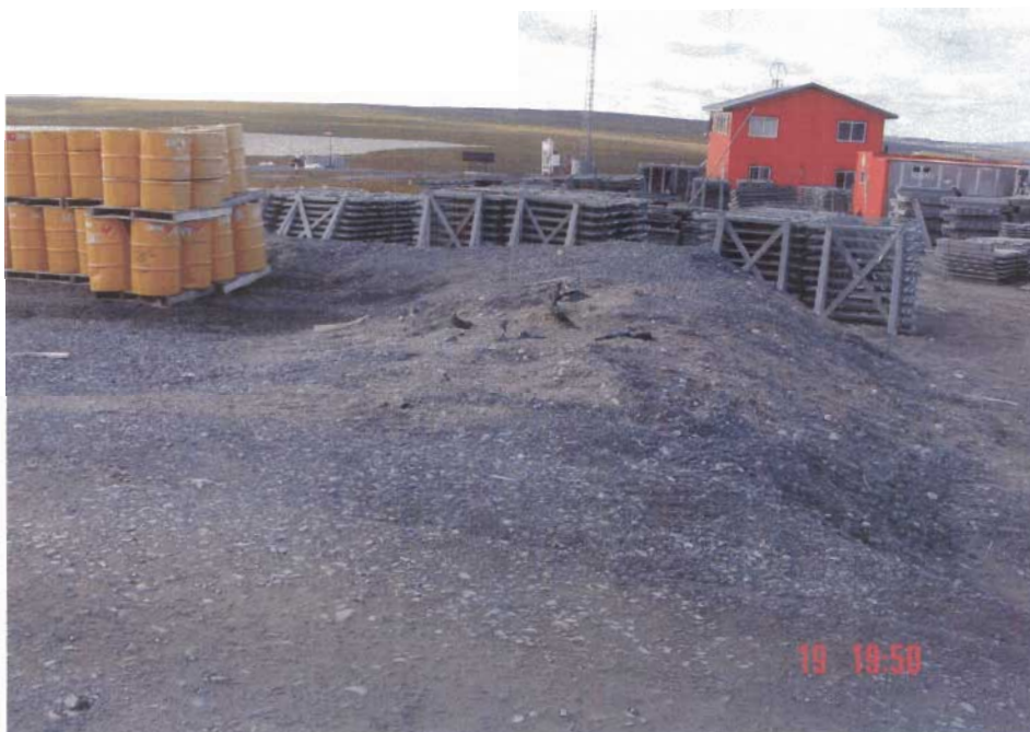
Photo # 6. Tank Farm and drummed fuel storage. The area is bermed and lined with synthetic impermeable liner.
