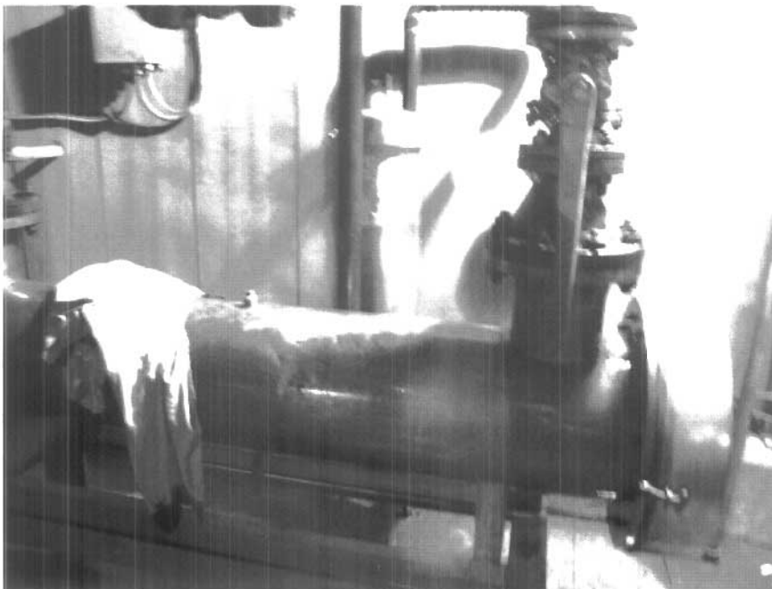
Figure 2. Ultraviolet Radiation Unit in the Water Treatment Plant at Lupin Mine.
