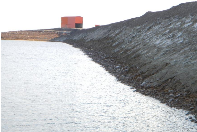
Undercutting in Dam K
