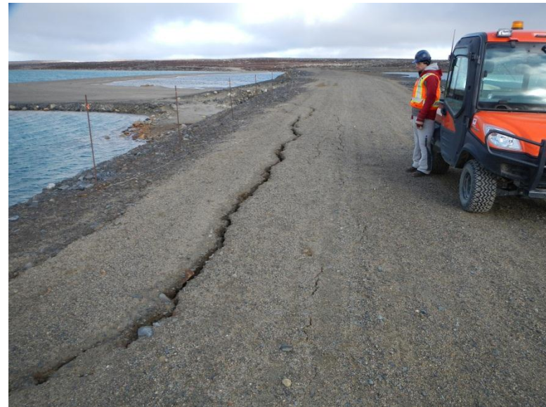
Tension Crack in Dam M
