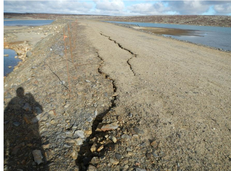
Tension Crack in Dam M
