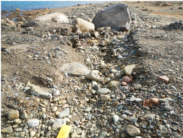
Breach in Dam L
