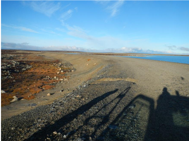
Erosion Gullies in Dam 4
