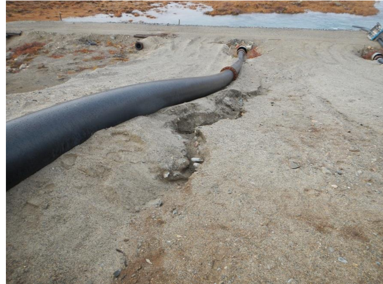
Erosion Gully in Dam 1A
