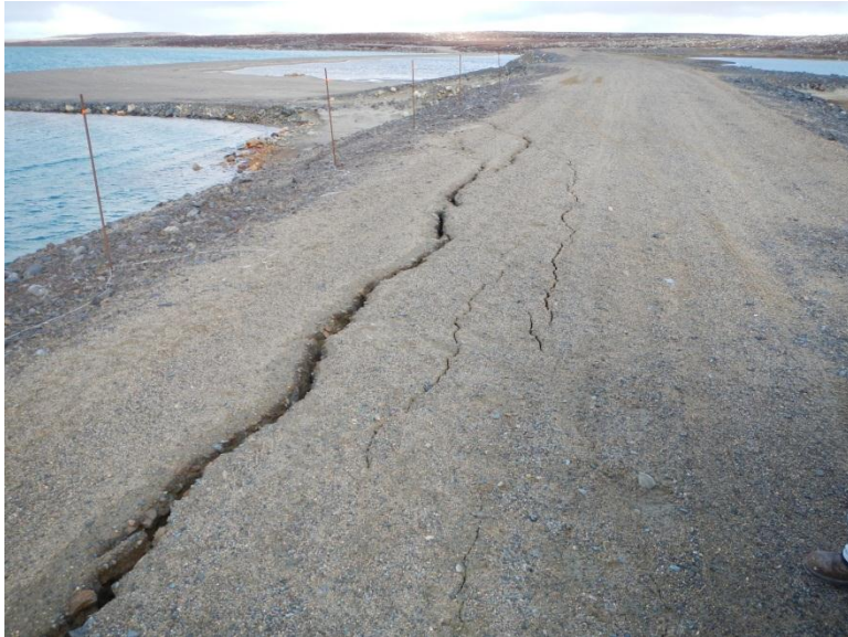
Tension Crack in Dam M
