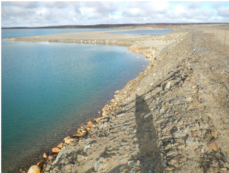
DS slope below Tension Crack in Dam 4
