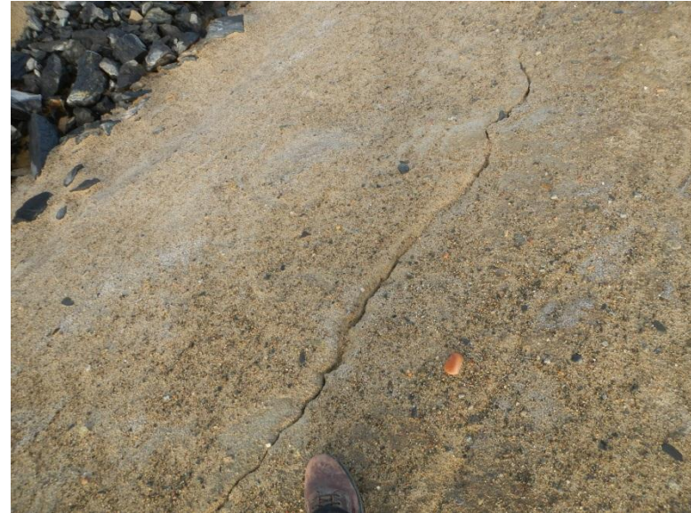
Minor Cracks in Dam 3
