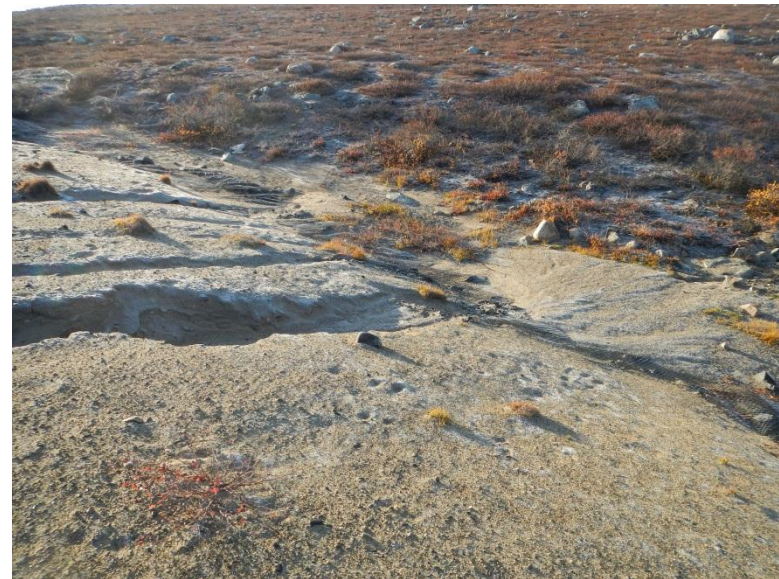
Erosion Gullies and Exposed Geogrid in Dam 4
