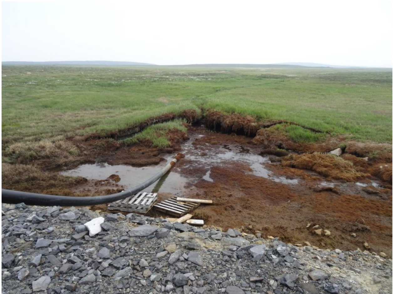
Figure 11. Permafrost degradation noted at discharge from LSL.
