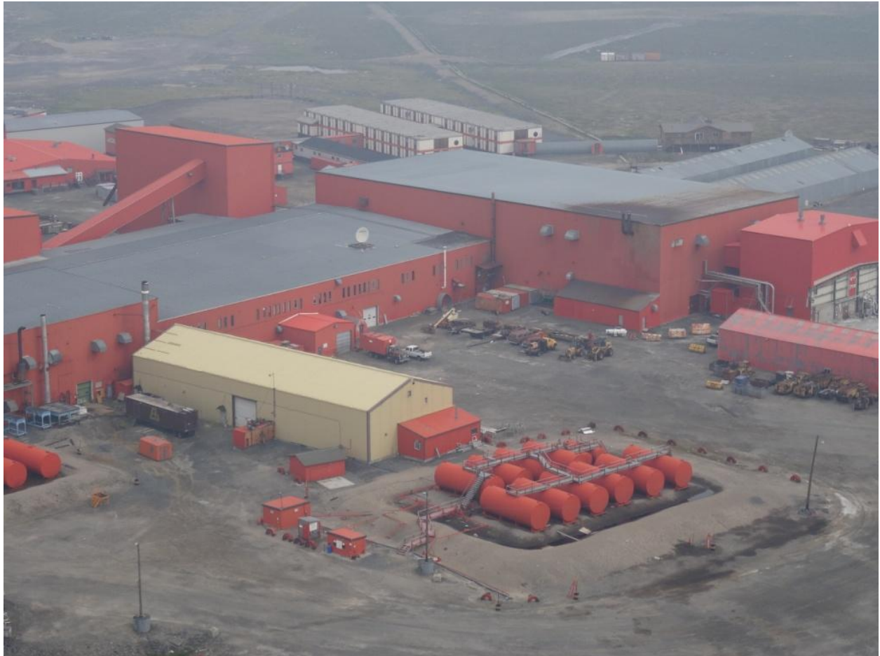
Figure 7. Satellite Tank (STF) Farm from the air. Heavy staining visible within and without.
