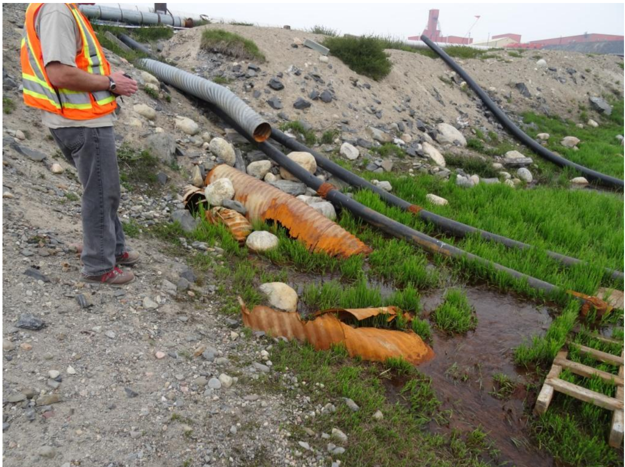
Figure 10. Steady flow seen through rusted culvert from the Upper Sewage Lagoon to the Lower Sewage Lagoon.
