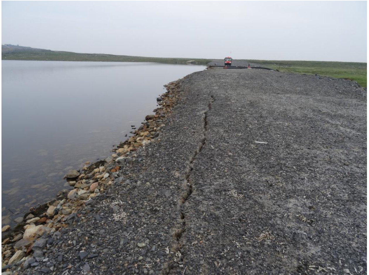
Figure 3. Crack in the dam at LSL.
