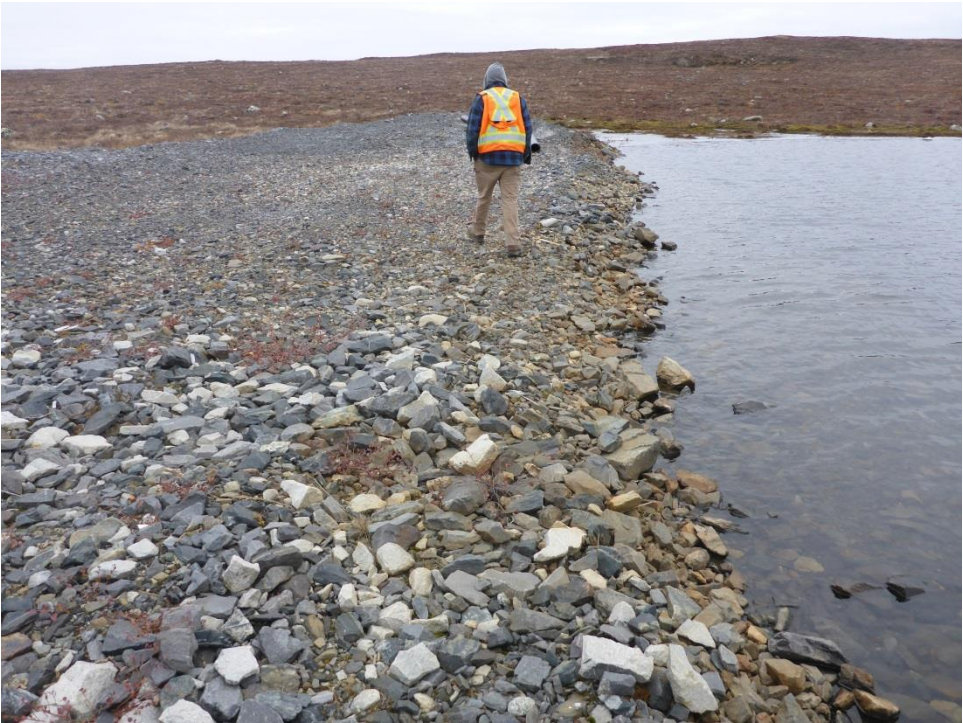
Photo 8: Looking southwest at low area of the Lower Sewage Dam toward the south abutment.
