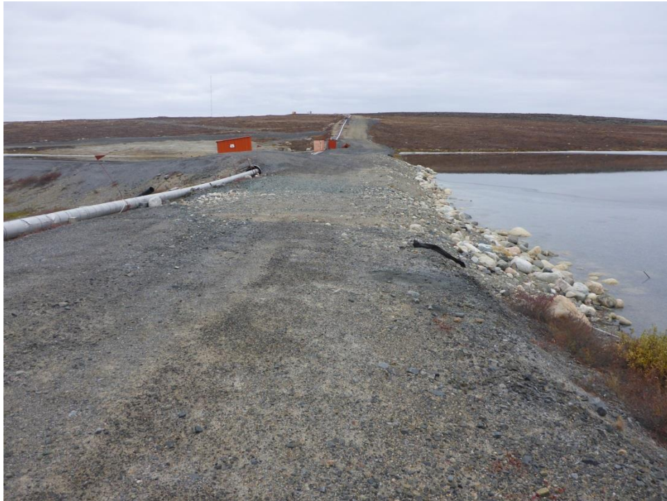
Photo 1: Looking southwest at the Upper Sewage Dam with the Upper Sewage Lake on the right.
