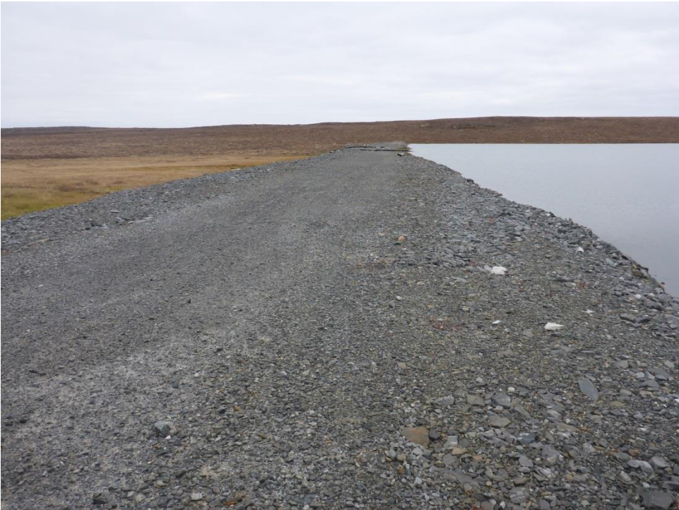
Photo 3: Looking southwest at the Lower Sewage Dam from the north abutment.
