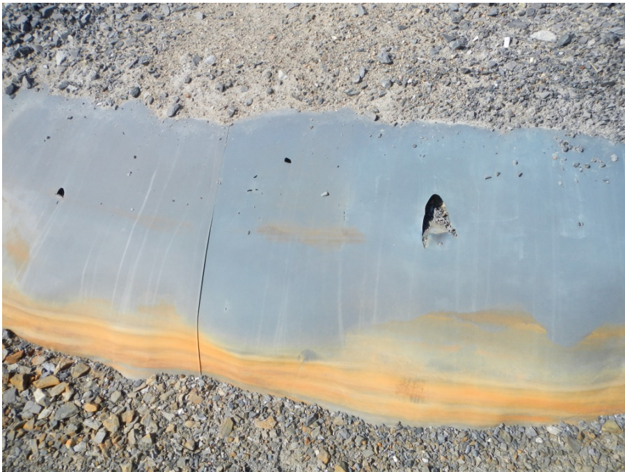
Picture 4: Closure up view of the damaged liner.
