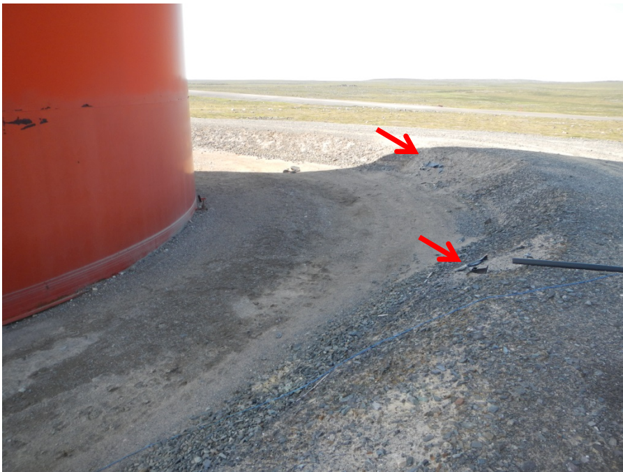
Picture 6: View of the damaged liner in the northwestern corner of the main tank farm.
