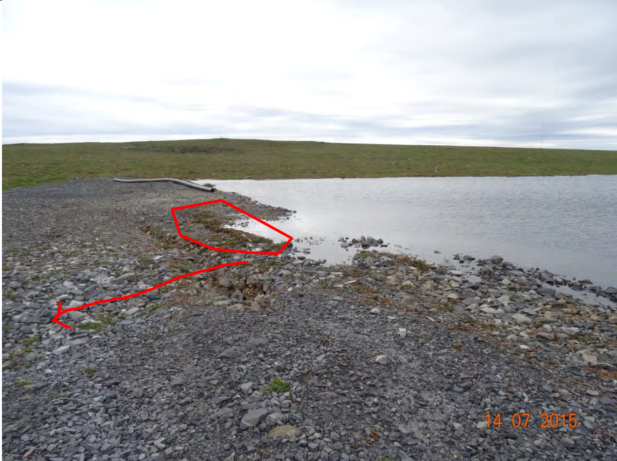
Description: Compromised section of Lower Sewage Dam. Effluent was trickling over this section at the time of the inspection in the direction of the arrow. It is suspected that the flow was greater prior to the inspection. Contents of LSL are pushed onto the berm (circled area).
