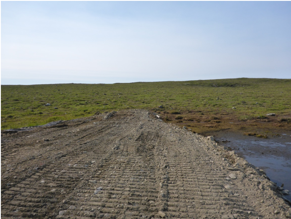
Photo 3: Looking south at the repair work complete on the southern abutment on the Lower Sewage Dam along the 2014 identified low area.
