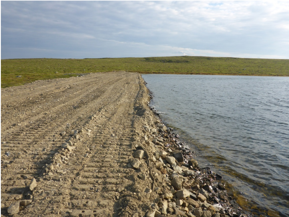
Photo 1: Looking south at the repair work complete on the upstream face on the Lower Sewage Dam along the 2014 identified southern area.
