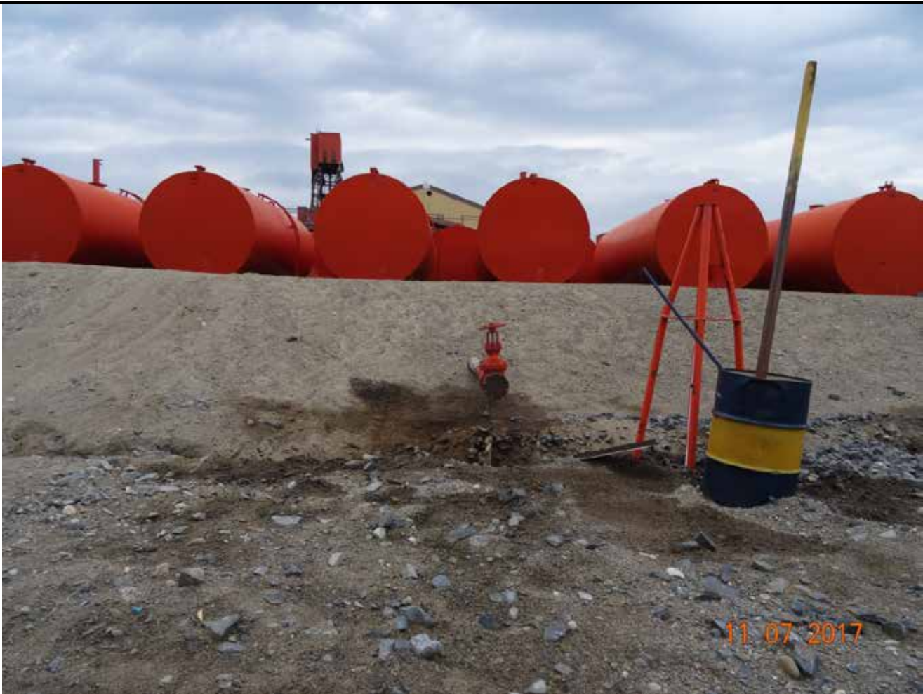
Description: Persistent staining at satellite tank farm.
