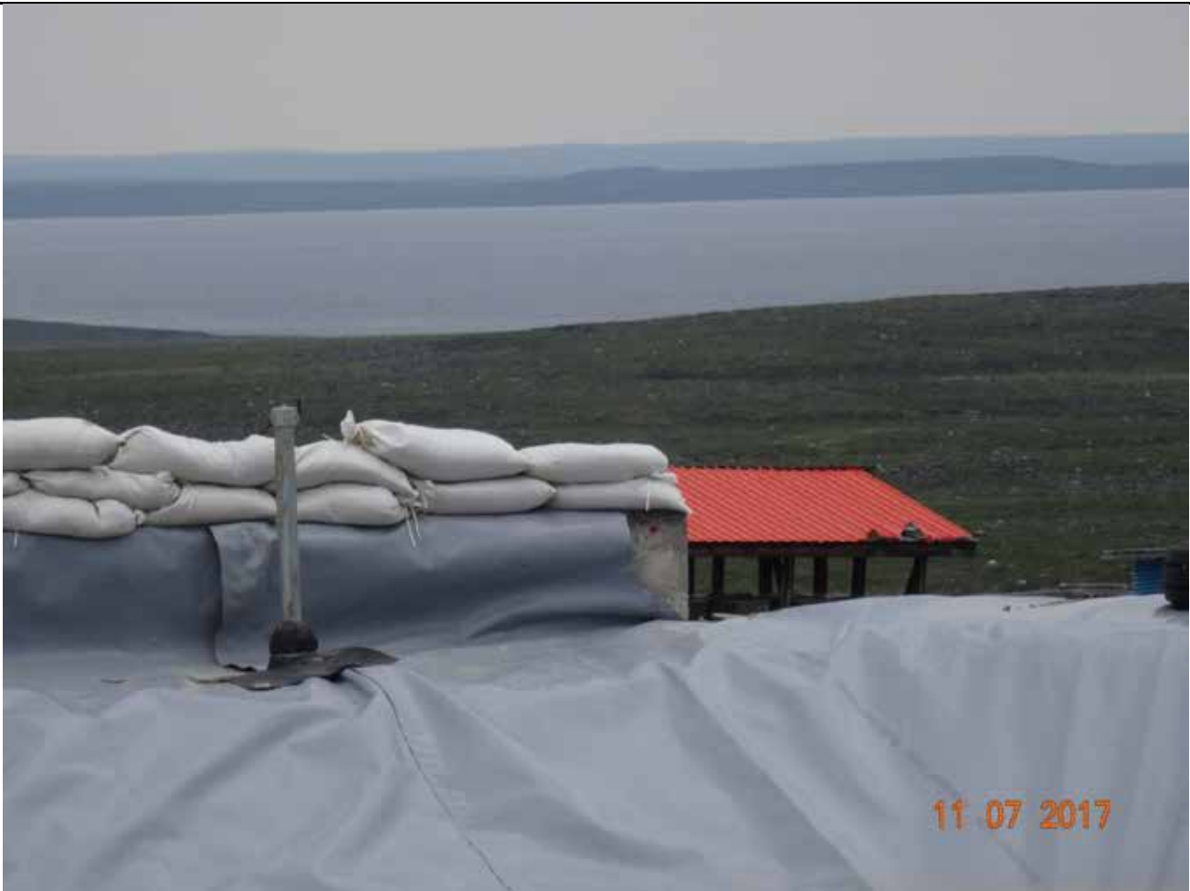
Description: Leak detection system built into landfarm.
