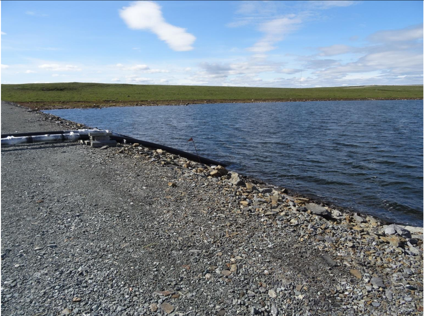
Description: Sewage Lagoon Pond showing Decant Intake Lines
