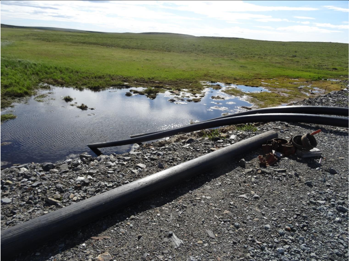
Description: Sewage Lagoon Pond showing Decant Outflow Lines
