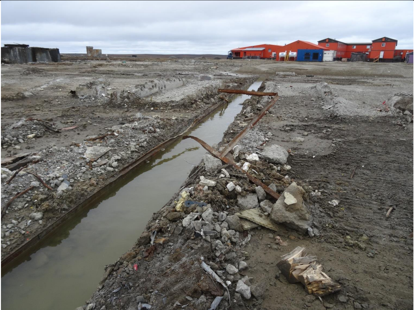
Description: #11 Mill, View 2 – Trench requires Draining and Cover Material
