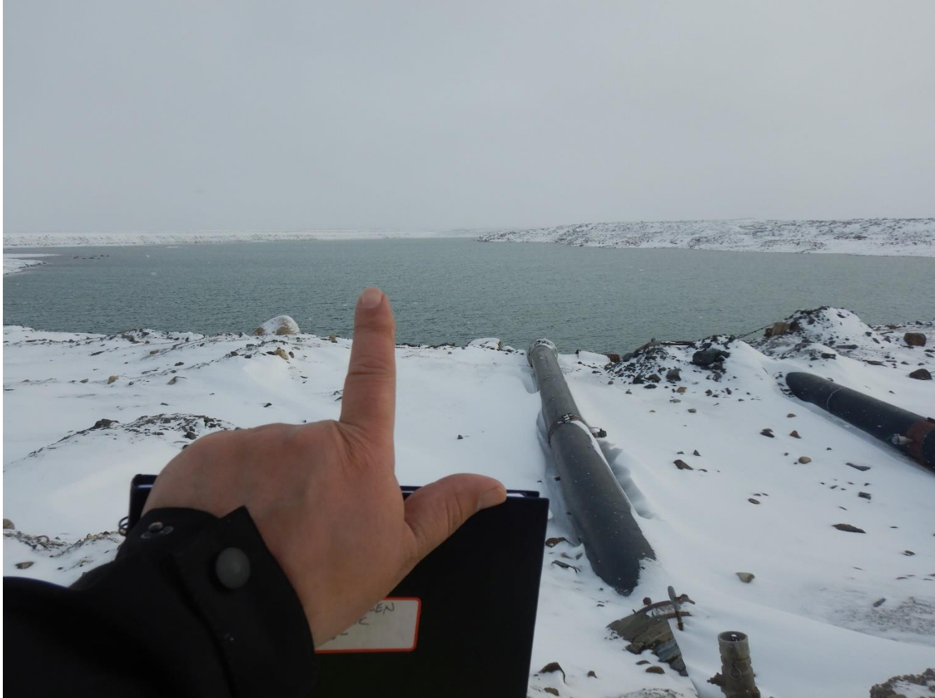
Description: Syphons over J-Dam from Pond 1 into Pond 2, View 1
