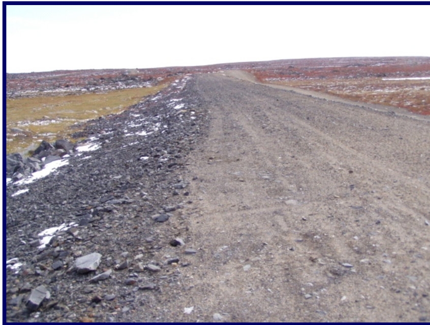
Photo 29 is a view of the crest on the upstream side. As previously noted, the riprap on the upstream side is relatively undulating. This dam does not currently retain any water.
