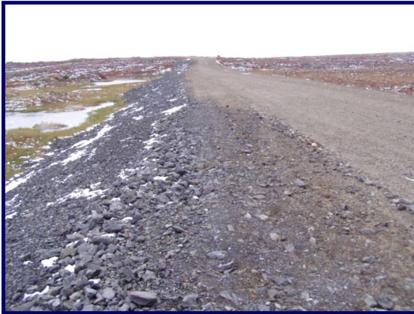
Photo 35 shows the upstream side and the crest. We do have a slight undulating nature to the riprap, likely a result of construction traffic activity.
