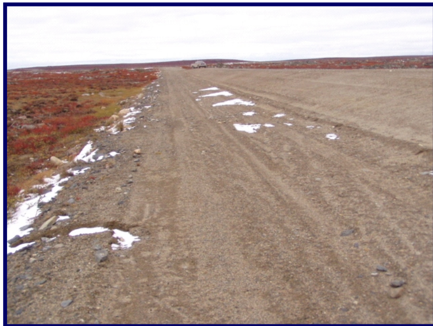
Photo 38 is a view along the access road toe berm. The downstream side has no signs of deformation or cracking from this perspective.
