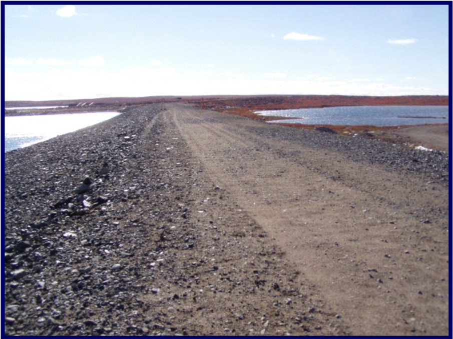
Photo 3 shows the condition of the crest looking towards the south. From this perspective, there are no signs of settlement or cracking.
