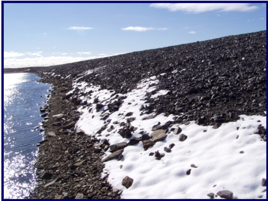
Photo 4 is a view of the upstream side. The distance from the current pond level to the crest is approximately 3.5 metres. Occasional small scarp form at the water level.
