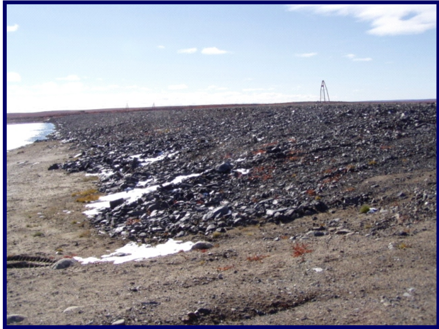
Photo 2 shows a view of the upstream side. The condition of the riprap appears to be satisfactory.
