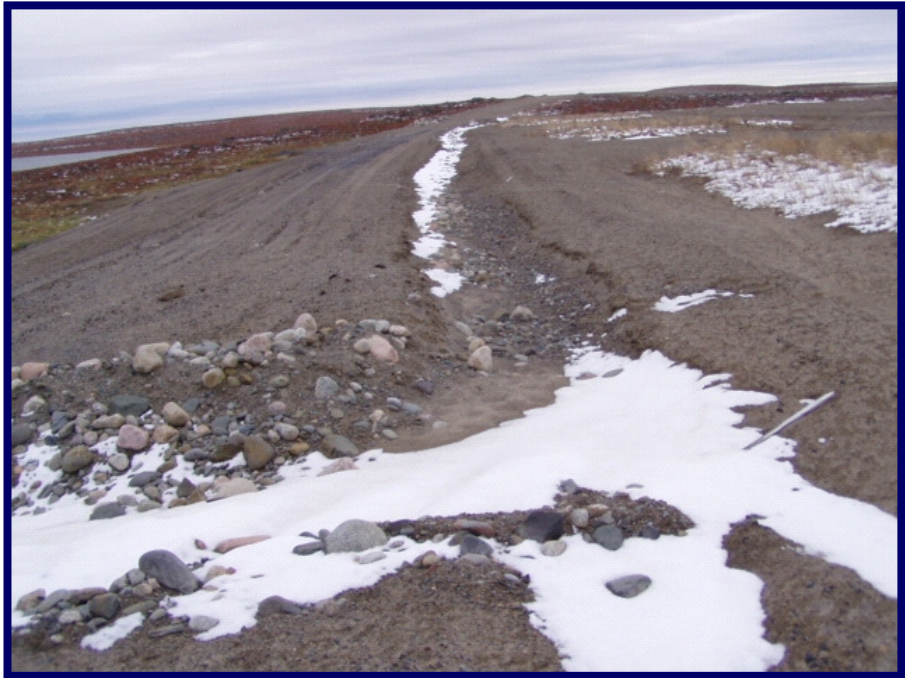
Photo 79 shows a small ditch which runs from the south end towards the north and then bends 90 degrees to the east across the crest of this dam. It is used to direct some of the surficial drainage and from this perspective, looks in satisfactory condition.
