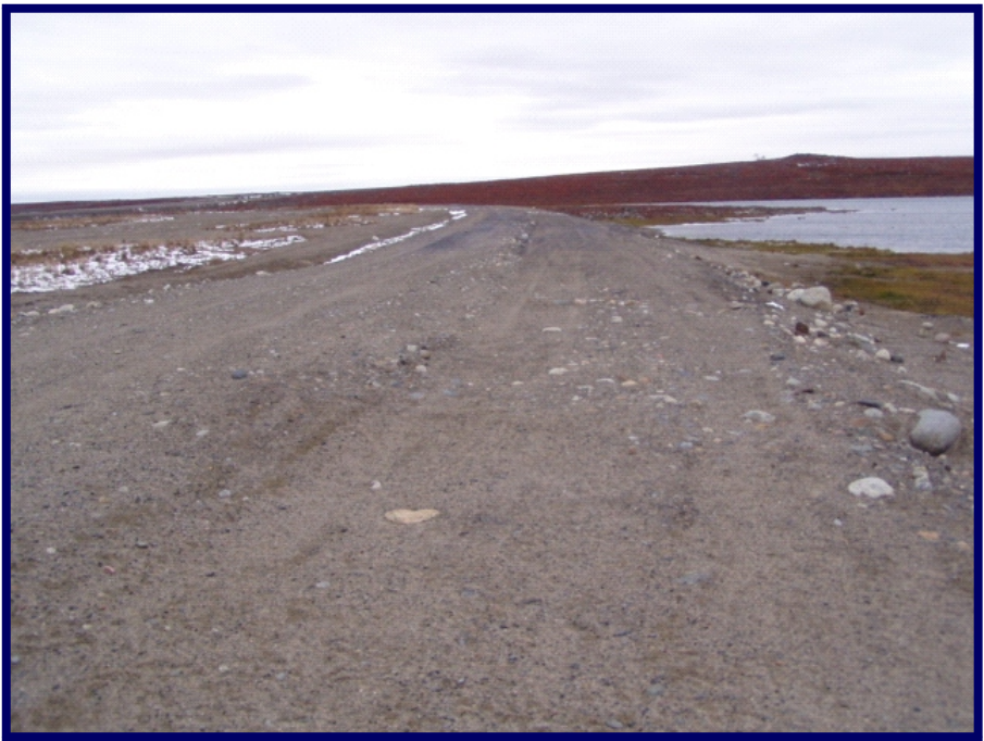
Photo 80 shows the condition of Dam 3 looking towards the north along the toe of this dam. There are no signs of significant erosion or any seepage discharging from this reclaimed dam.
