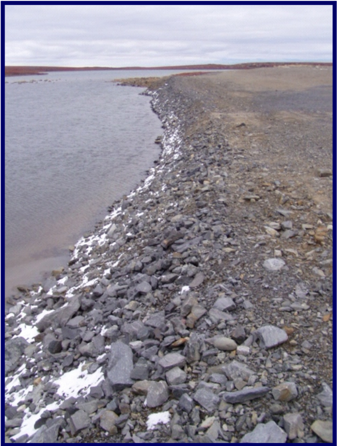
Photo 73 shows the toe edge where it meets Boomerang Lake. This is the area where historically cracking has been seen, No significant sloughs are noted right now.
