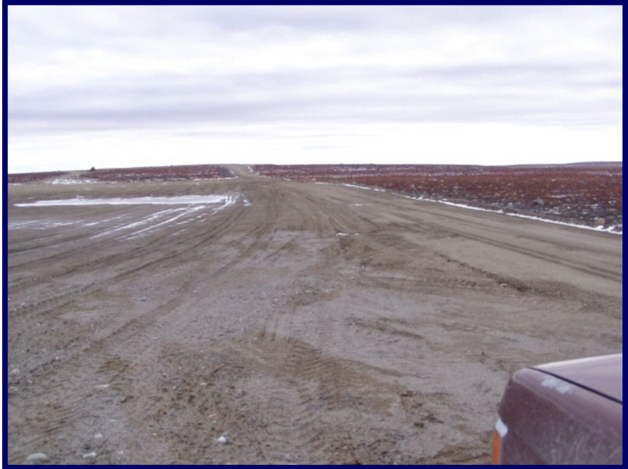
Photo 41 shows the crest of Dam 6 looking towards the south abutment. As can be seen, reclamation and placement of cover has occurred on the upstream side hence, covering over the majority of the tailings.
