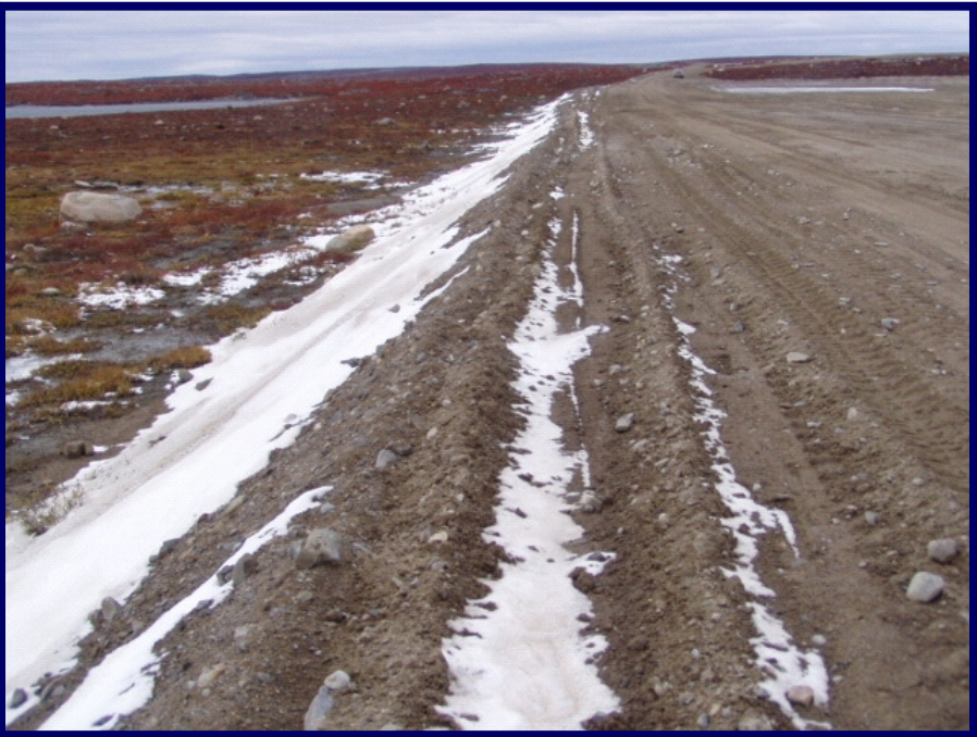
Photo 47 shows a view of the downstream toe looking towards the north. Construction traffic has caused a number of ruts and pushed up some windrows on the toe crest.
