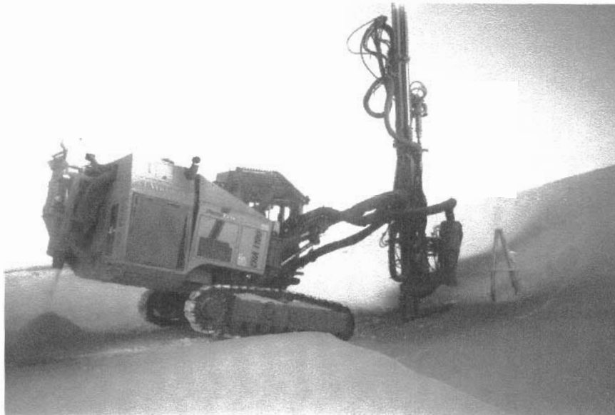
Photo 1 - Drilling at downstream toe of Dam 2
