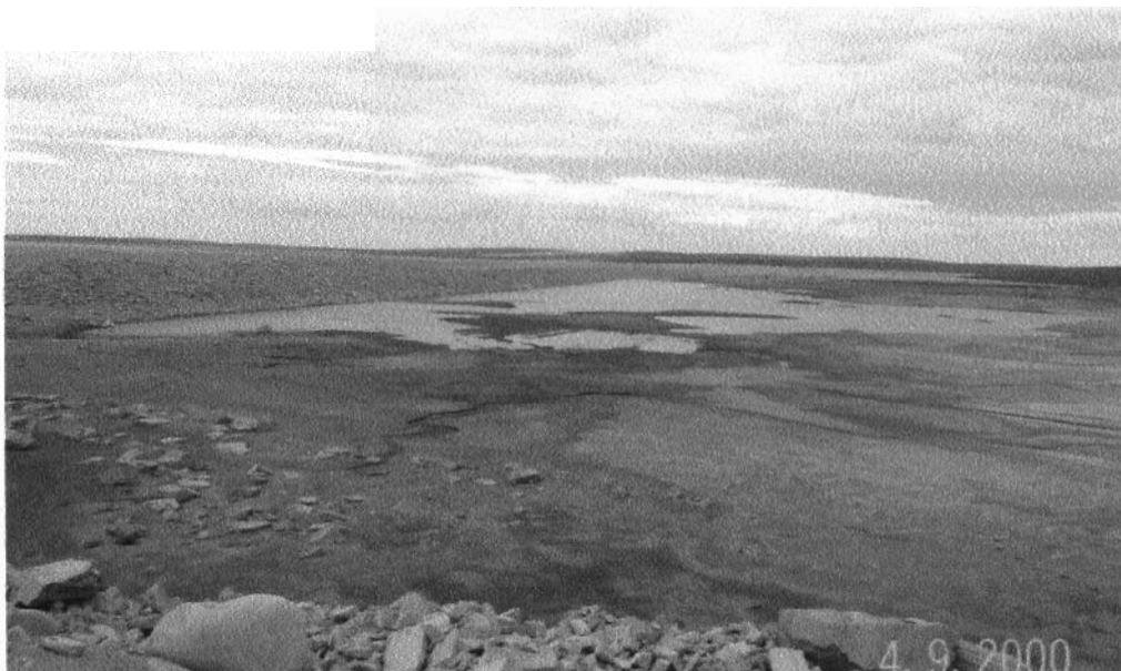
Photo No.2 Lupin Tailings Containment Area - Mdam construction; September 2000
