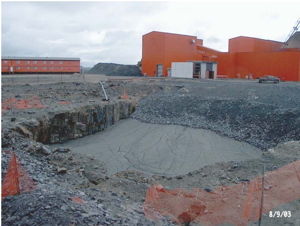
Photo 3 – Waste rock cap placed on paste filled stope.
