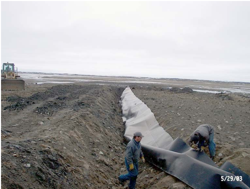
Photo 8 – Installing liner in Cell 1 test pad
