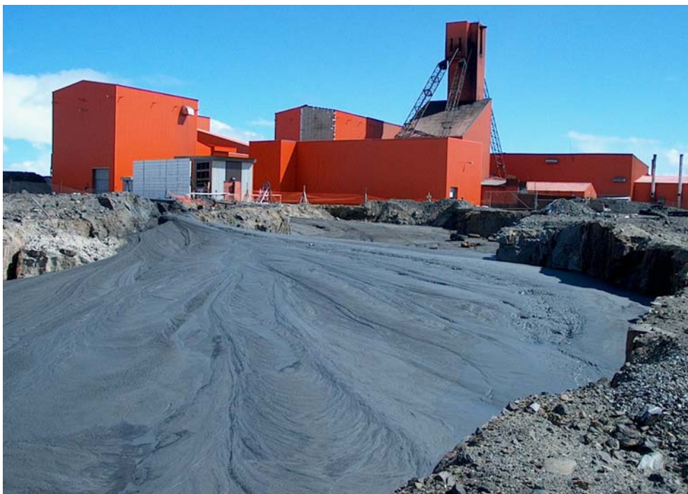
Photo 2 – Paste backfill being poured into Centre Zone crown pillar stope. View to south.
