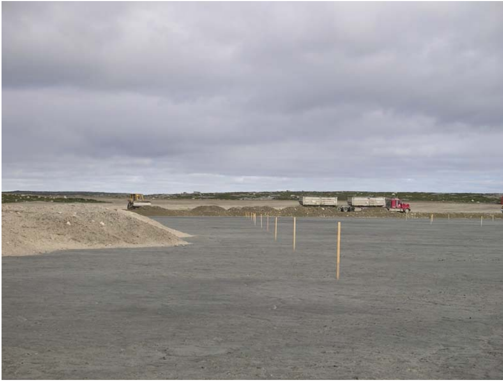
Photo 7 – Placing esker cover on Cell 3. Stakes are 1 metre high.
