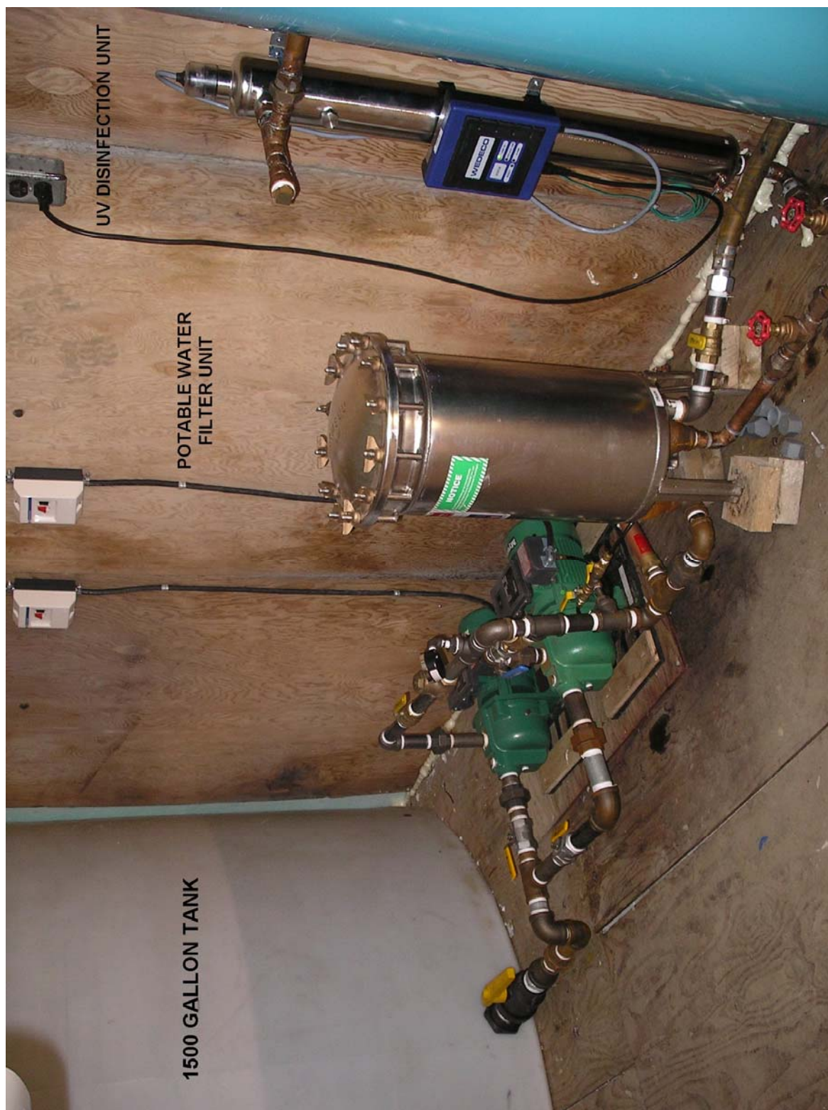
Photo 2 – Water storage tank, potable water filter unit, UV unit. August, 2006.
