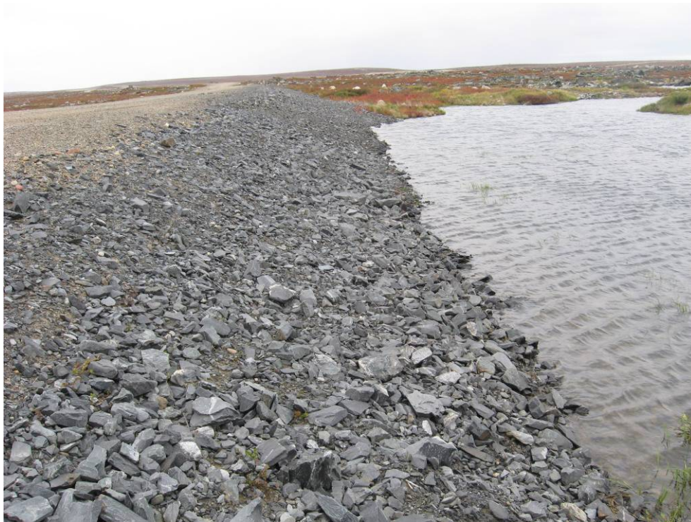
Dam 1C: Upstream
