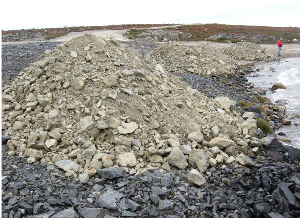
Dam 2: Upstream – New Riprap Material
