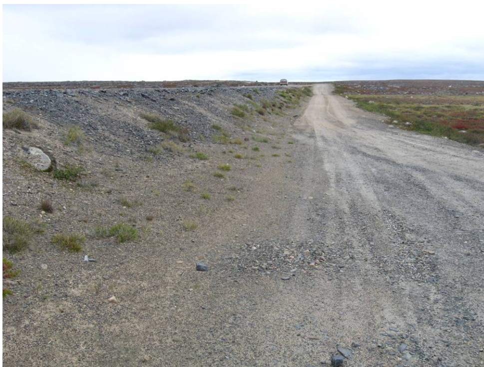
Dam 1B: Downstream
