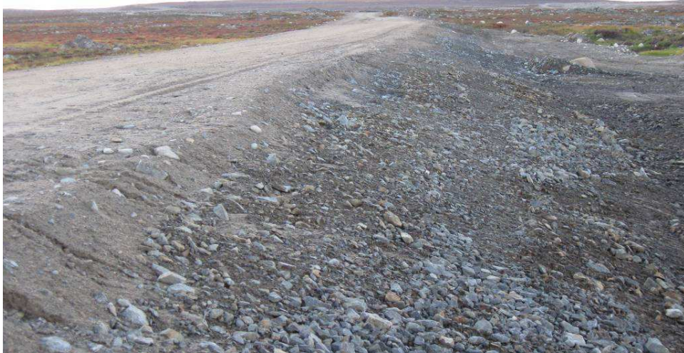
Dam 1C: Upstream (Minor Erosion Gullies on Shoulder of Granular Surfacing)
