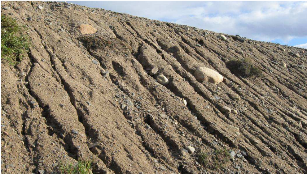
Dam 2: Downstream Slope Erosion Gullies and Rills
