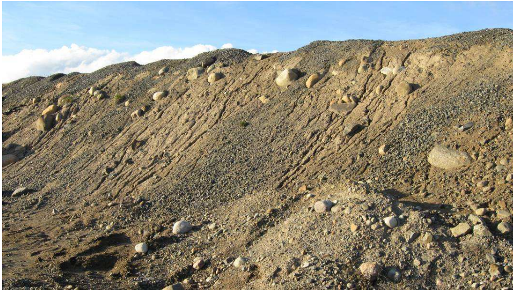
Dam 1A – Downstream Slope (south side of Siphons) Erosion Gullies
