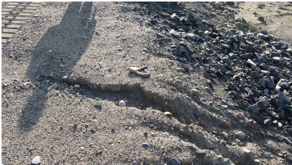
Dam 5: Downstream. Erosion gullies.
