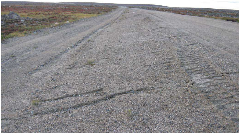
Dam 1C: Downstream Slope (Some Minor Erosion Gullies)
