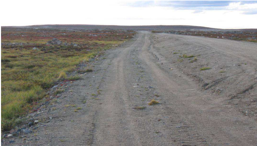
Dam 1C: Downstream Slope (Some Minor Erosion Gullies)
