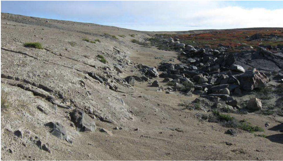
Dam 4: Downstream slope, east of cofferdam. Extensive erosion gullies (exposed geogrid).
