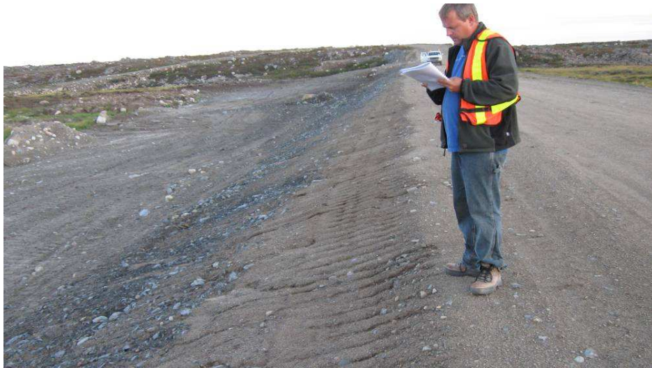
Dam 1C: Upstream (Minor Erosion Gullies on Shoulder of Granular Surfacing) Souther 2/3 of Upstream Slope Has Been Regraded/Extended with a Mixture of Rip Rap and Esker Material
