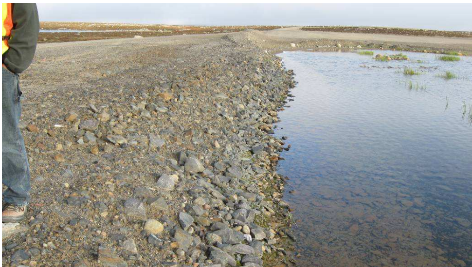
Dam 6: Upstream. Riprap in area of small pond.
