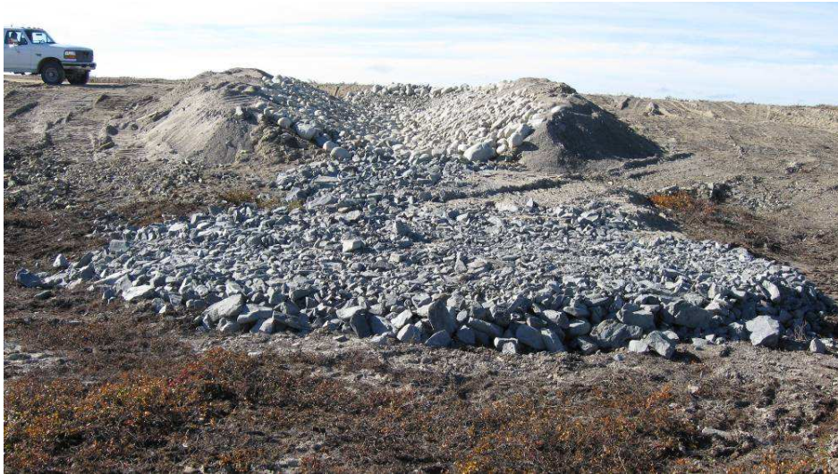
Dam 3: Downstream side of spillway (splash pad). Spillway side slope constructed at about 2.5H:1V (steeper than 3H:1V specified). Slopes on the outside of the spillway channel are also steeper than specified.
