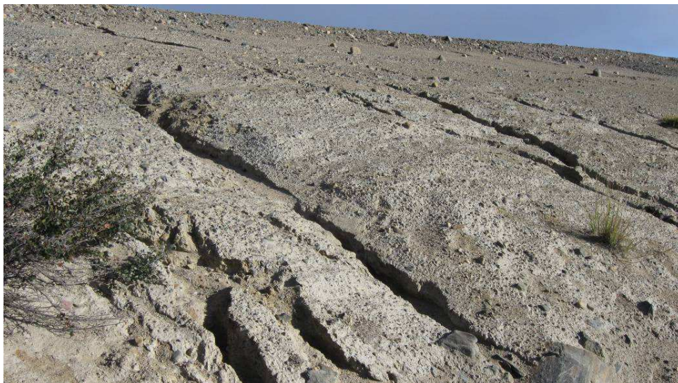
Dam 4: Downstream slope, east of cofferdam. Extensive erosion gullies
