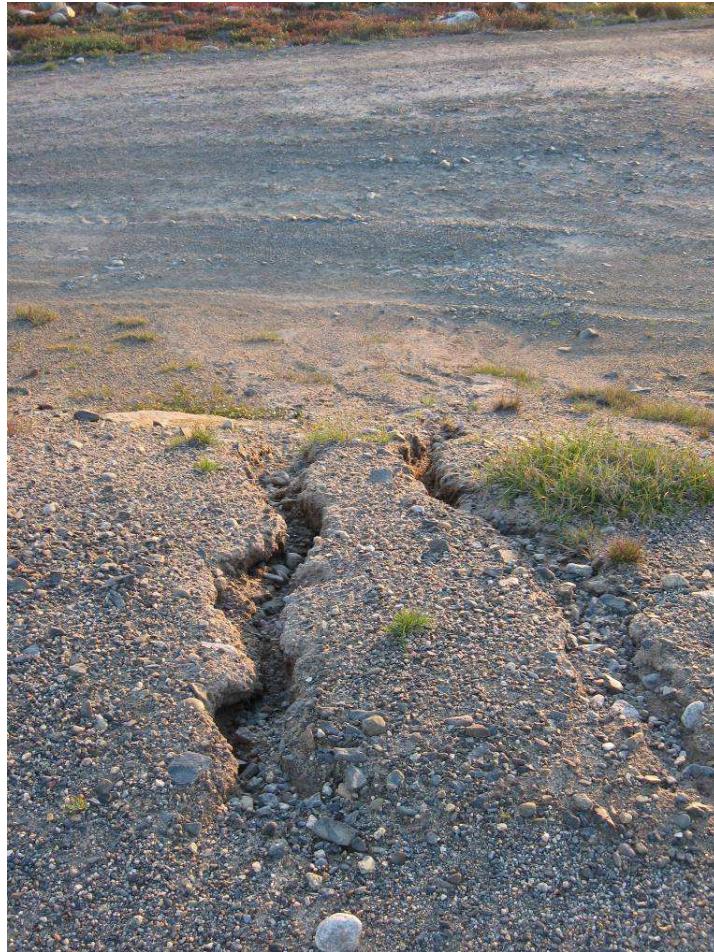
Dwonstream Slope: Erosion Gullies
