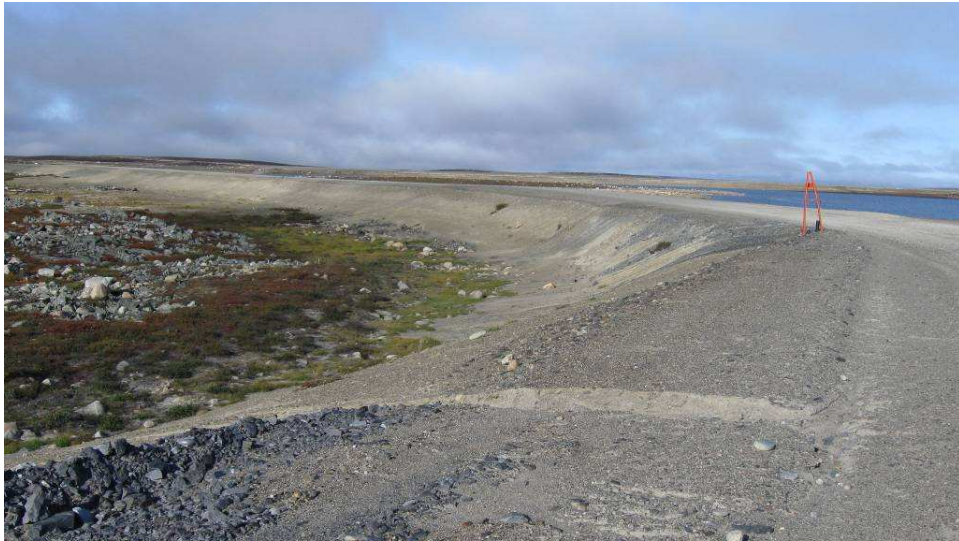
Dam 4: Downstream slope, east of cofferdam (looking west). Extensive erosion gullies
