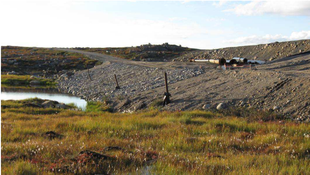
Dam 1A: Downstream Access Road toe Berm Looking North (Note, Downstream Slope Regraded and Covered with Riprap in 2010).
