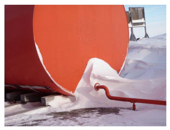
Photo 5: M-22 Disconnected From Piping, Feb 2012.
