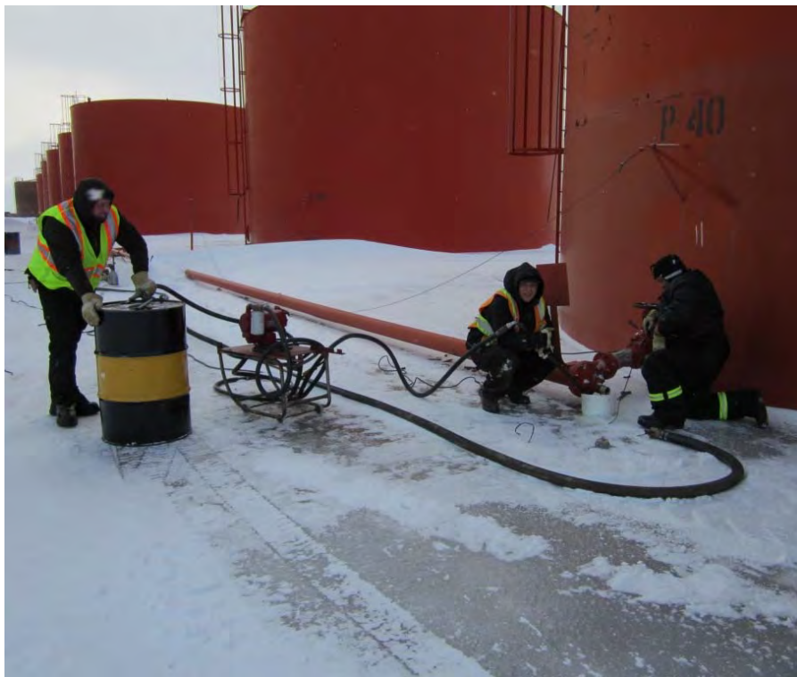
Photo 25: Remedial Works in MTF, Oct 2011.
