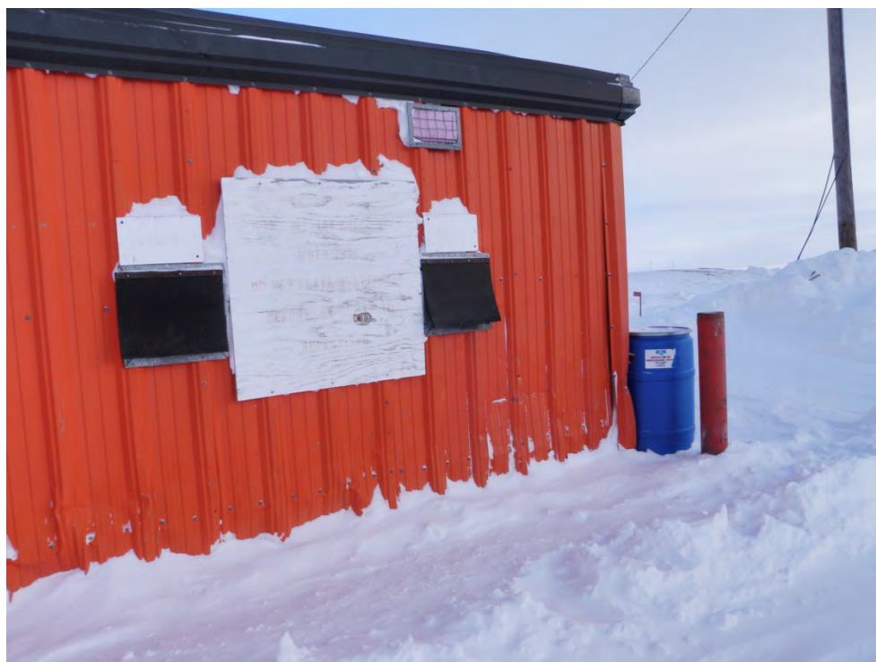
Photo 8: Diesel Dispensing Station, STF, Feb 2012.
