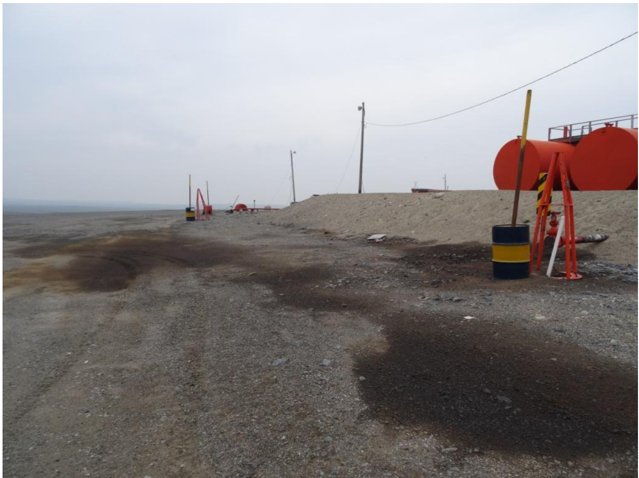
Figure 8. Staining outside the STF berm.
