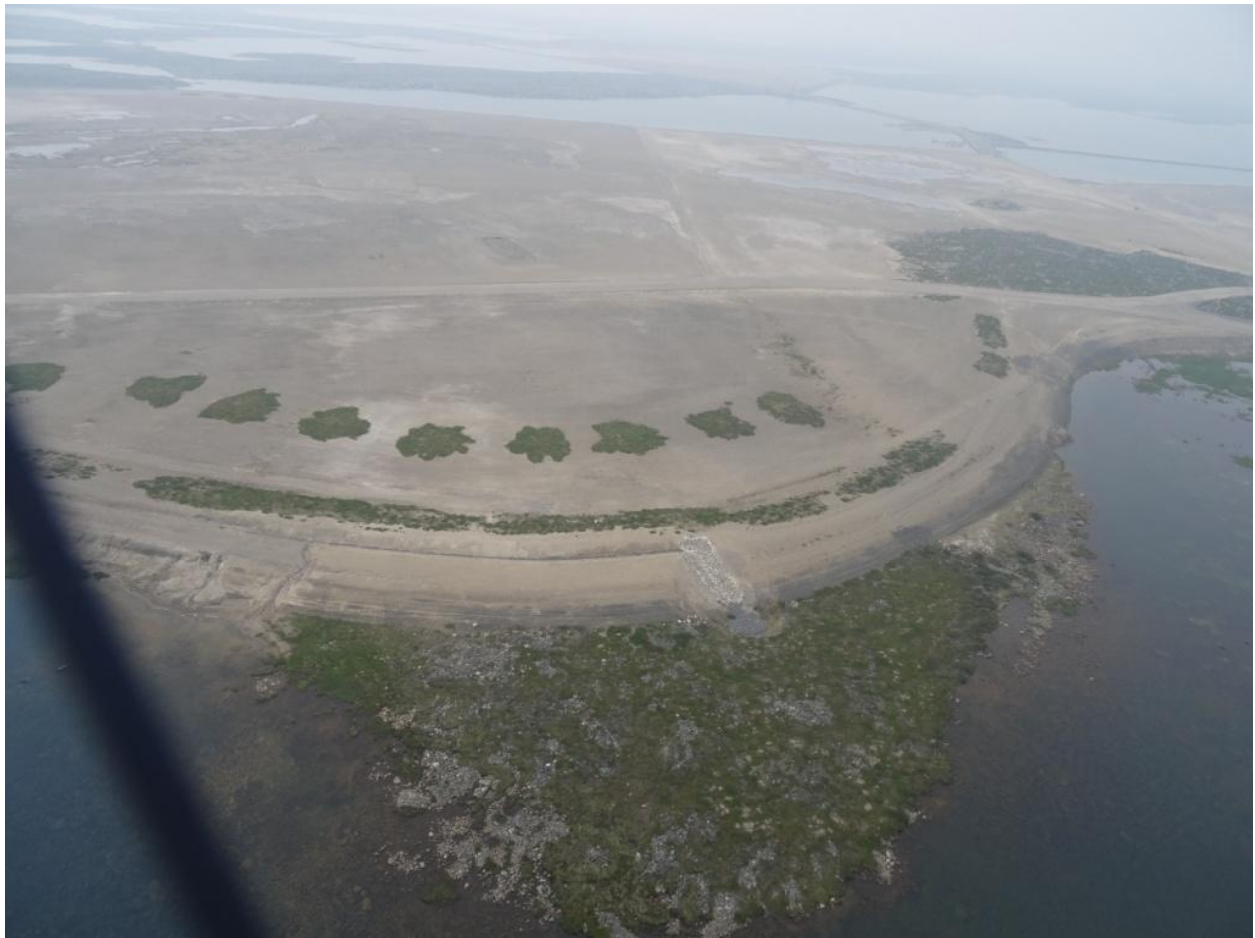
Figure 17. Growing vegetation cover near Dam 6. Recurring washouts also visible on left, resulting in deposit to water.
