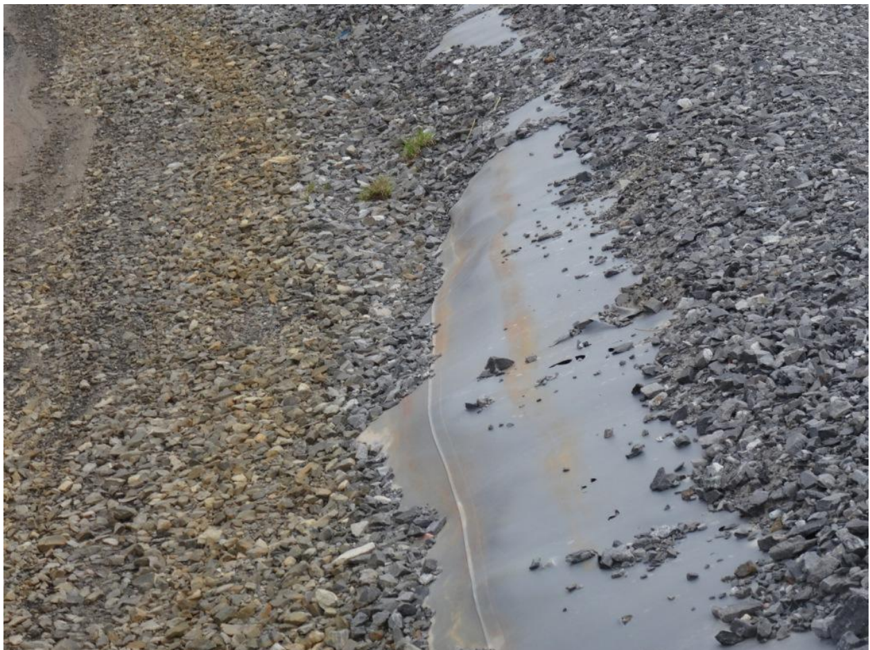
Figure 6. Rips visible in the exposed liner at the MTF.
