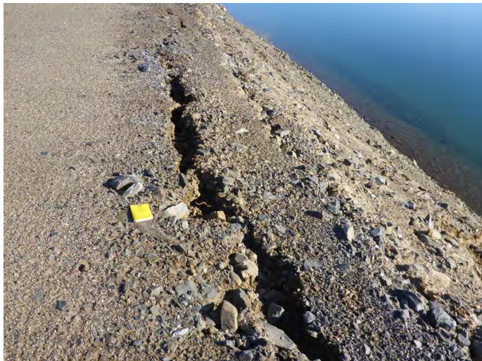
Photo 34: Close up view of the new tension cracks observed in 2014, in face of the dam toward Pond 1.
