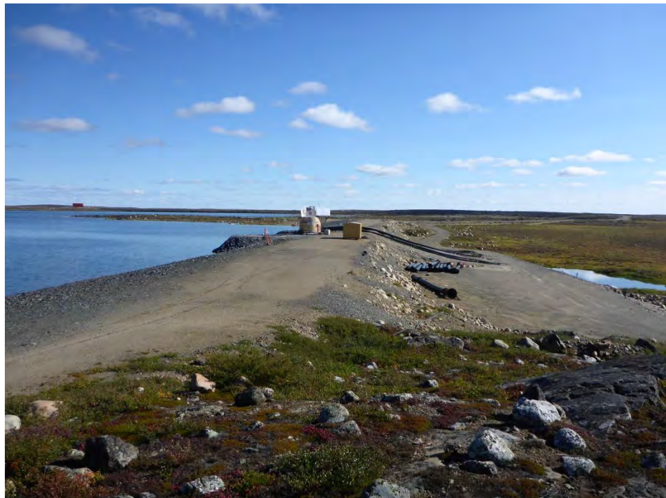
Photo 4: Looking south at Dam 1 A
