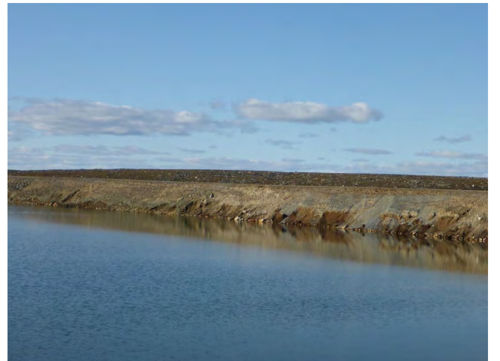
Photo 36: Looking northeast of at the Dam M facing toward pond 2. Note the failure surfaces at the toe.
