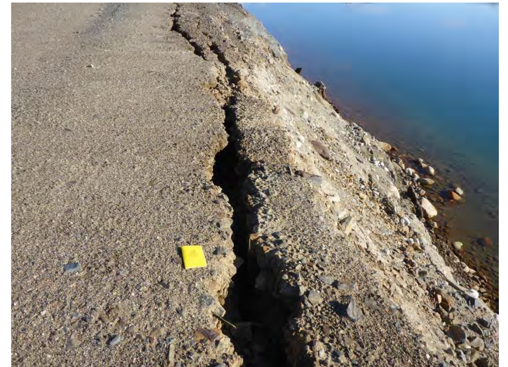
Photo 33: Close up view of the new tension cracks observed in 2014, in face of the dam toward Pond 1, upwards of 0.3m wide and 0.5m deep.
