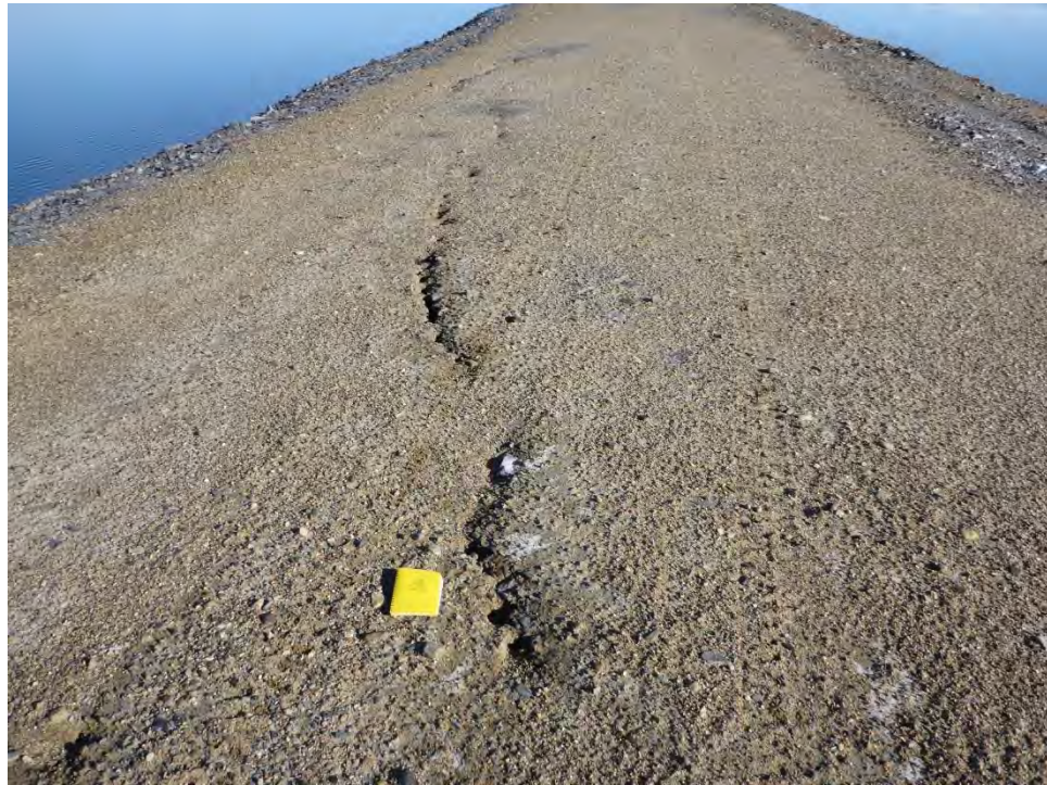
Photo 31: Close up view of the new tension cracks observed in 2014, through the centerline of the dam.
