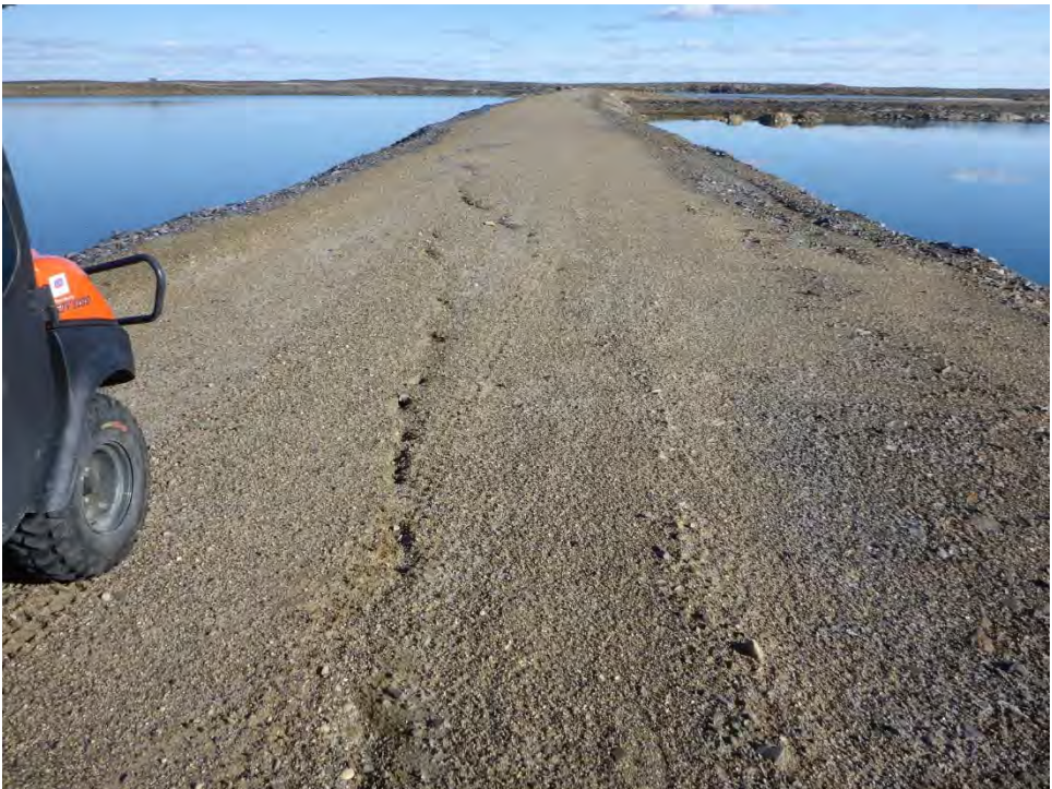
Photo 30: Looking southeast at the new tension cracks observed in 2014 on Dam M with Dam J in the left background.
