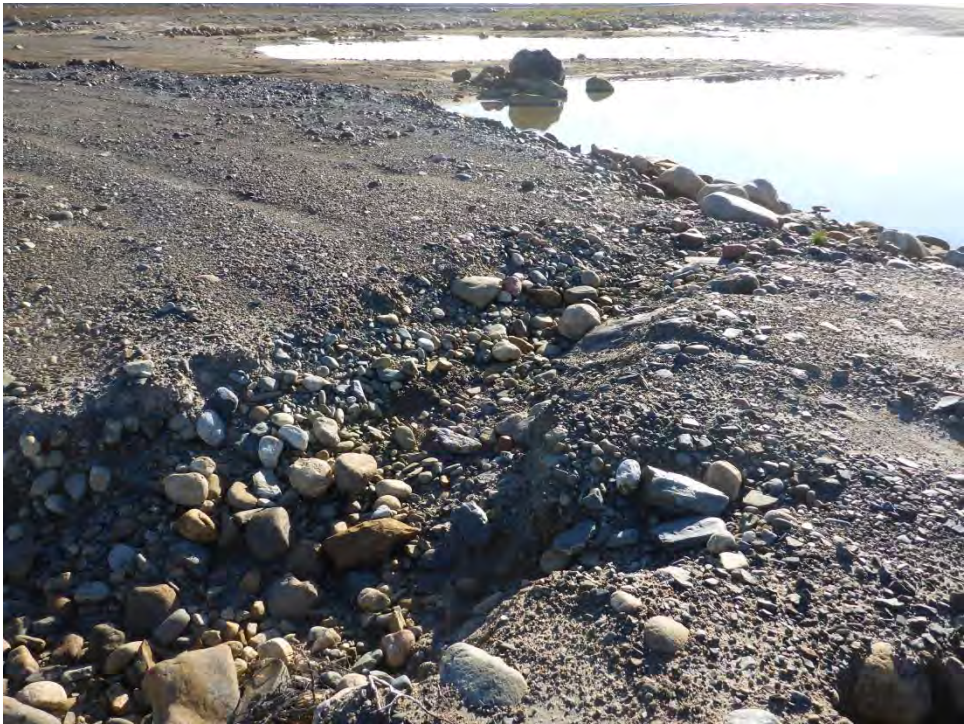
Photo 44: View of erosion channel near the south abutment of Dam L with Cell in the background.
