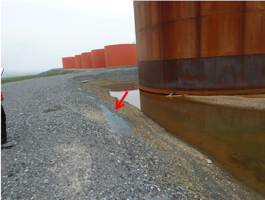
Picture 3: North view from the back of the tank farm with shallow ponding water. Note the exposed and damaged liner.
