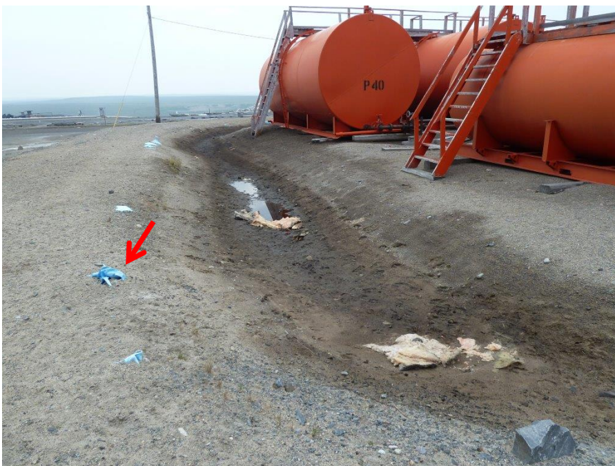
Picture 8: South view of the eastern embankment of the satellite tank farm with exposed and damaged liner.
