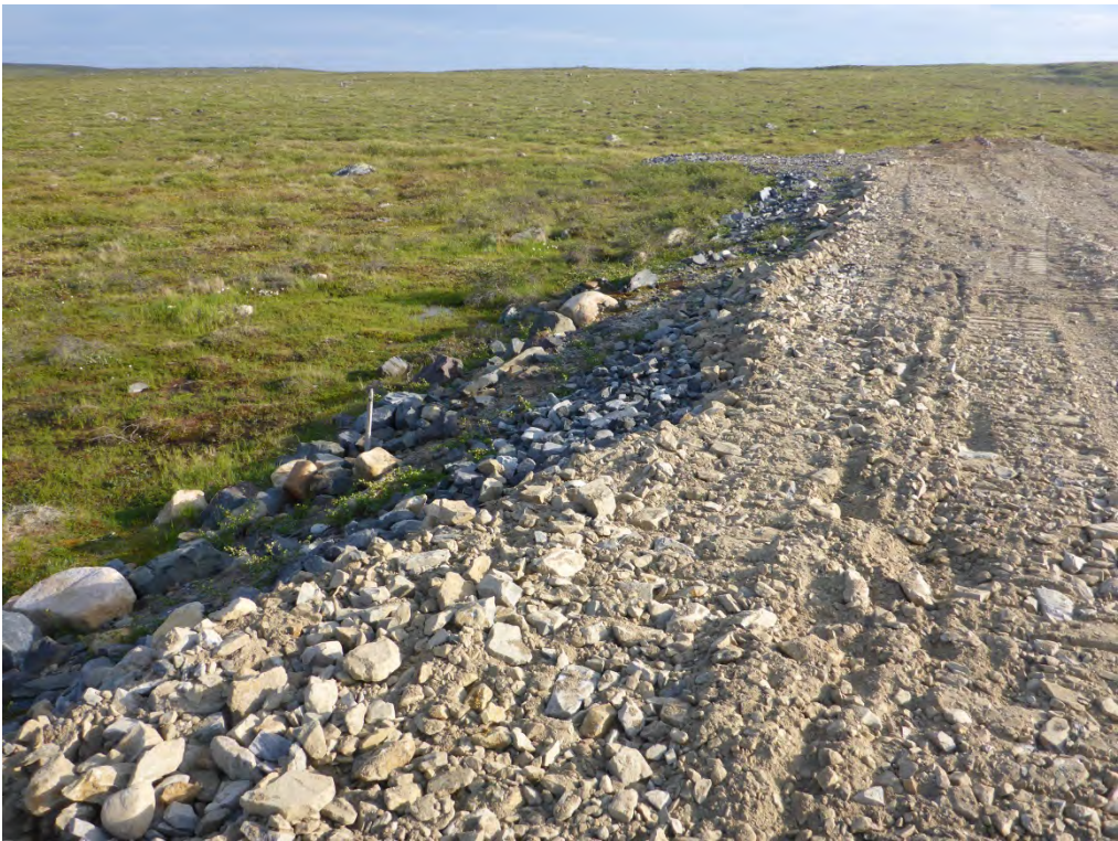
Photo 2: Looking south at the repair work complete on the downstream face on the Lower Sewage Dam along the 2014 identified southern area.
