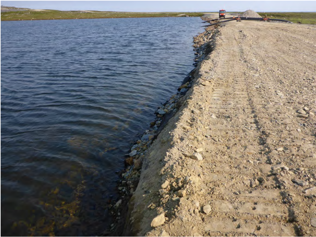
Photo 4: Looking north at the repair work complete on the upstream face on the Lower Sewage Dam. Note the siphons in background actively lowering the water level.
