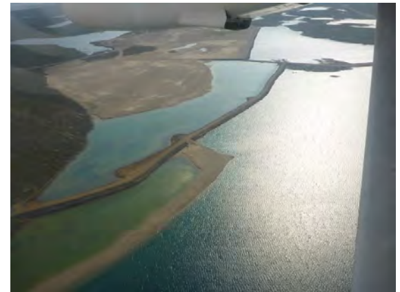
Photo 45: Aerial view of Dam N. Note the near submergence due to the high water level in Pond 2 during the time of visit.
