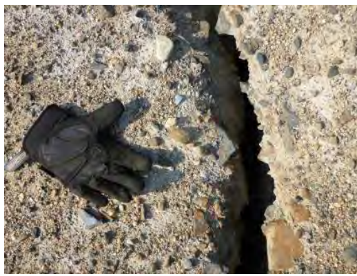
Photo 29: Close up view of the original tension cracks on Dam M.
