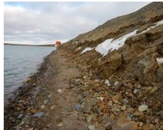
Photo 47: Picture taken on October 6 th at Dam L showing the armored toe that was previously submerged in Pond 2.
