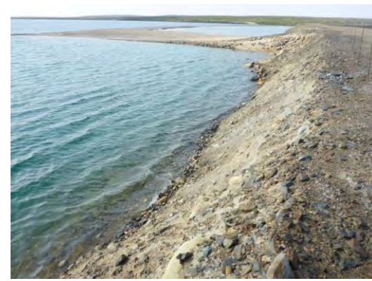
Photo 30: Looking northwest on Dam M at the over steepen slope directly downstream of the cracks, with Dam N and Pond 2 to the left.
