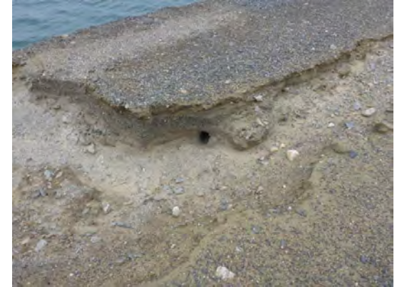
Photo 21: Close up of erosion gully in Dam 4, the burrow from ground animal.
