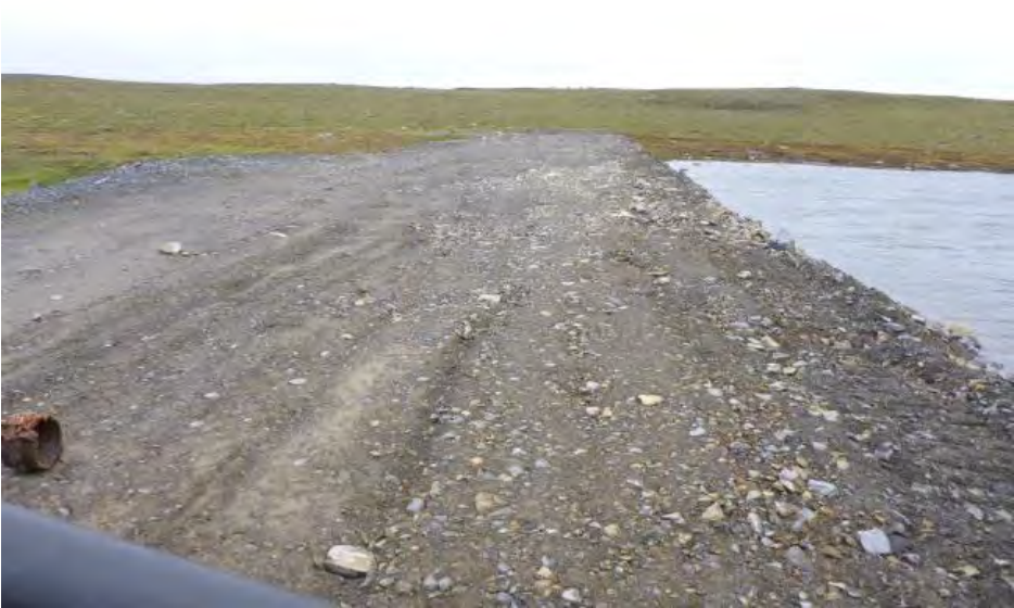
Photo 2: Looking south at the Lower Sewage Dam southern abutment on the additional fill placed to raise the elevation.
