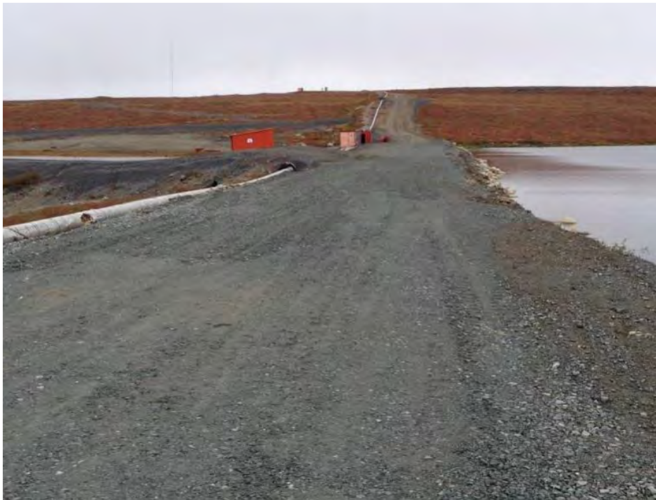
Photo 4: Looking south from the Upper Sewage Dam north abutment on the repaired crest with additional fill placement.
