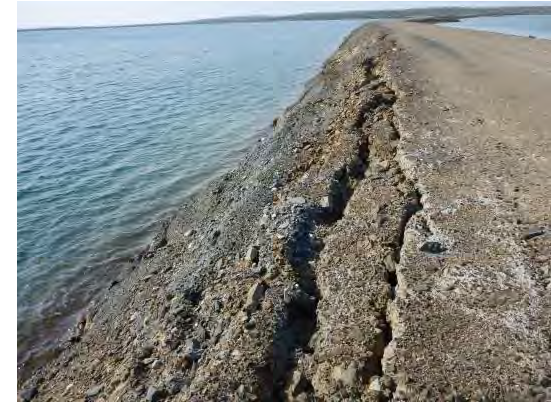
Photo 33: Close up western view of Dam M the new tension cracks observed in 2014, in face of the dam toward Pond 1, upwards of 0.3m wide and 0.5m deep.
