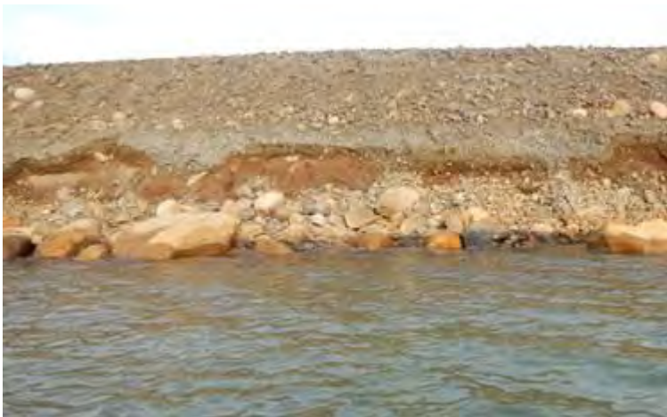
Photo 46: Picture taken on October 6 th at Dam M showing the armored toe that was previously submerged in Pond 2.
