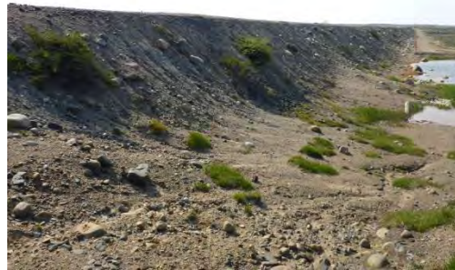
Photo 2: Looking south at the seepage collection ponds at toe of Dam 2.
