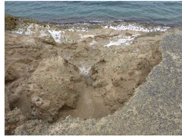
Photo 32: Looking northwest, down toward the toe at one of the five erosion gullies along the upstream crest of Dam K
