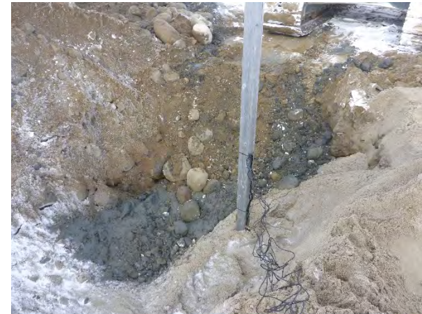
Photo 40: Installation of the sensor string at the tailings and cover contact, 1m below cover surface.
