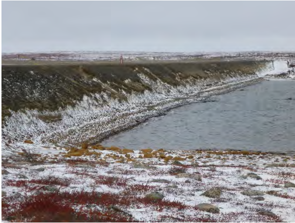
Photo 31: Looking southwest from the east abutment of the eroded toe at Dam K
