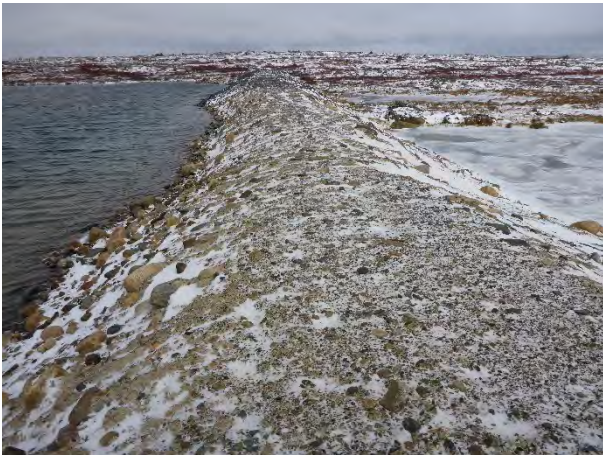
Photo 50: Looking north at the eroded crest slopes and sloughed crest of northern divider dyke.
