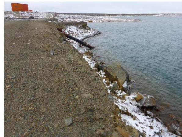
Photo 27: Looking south at the eroded downstream slope of Dam J.
