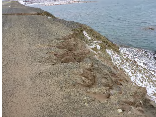
Photo 34: Looking southwest from near the east abutment along the downstream crest of Dam K at the erosion gullies.
