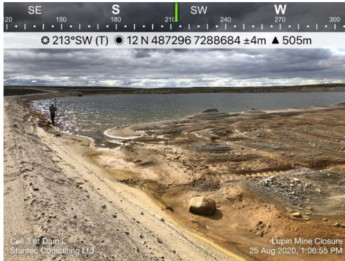
Photo 38: Looking southwest at the upstream slop of raised Dam L and cover construction in the ponded area of Cell 3.
