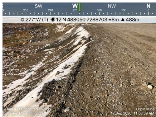
Photo 19: Looking west at a repaired erosion gully at the downstream crest near the east abutment of Dam 4.
