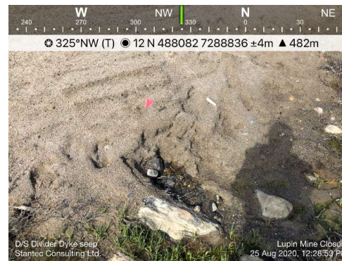
Photo 52: Looking northwest at one of the seepage zone at the toe.
