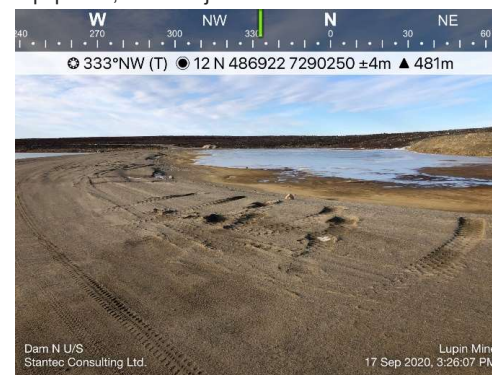
Photo 49: Looking north at the crest of Dam N and ponding water with approximately 0.8m freeboard.
