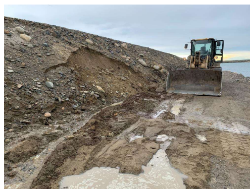
Photo 47: Looking at localized failure caused by the equipment near the junction of Dam N
