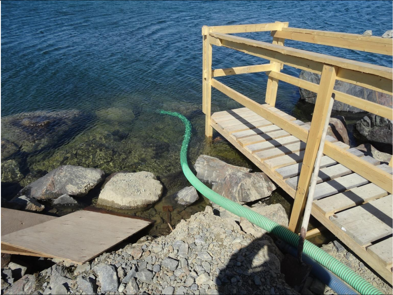
Description: Water Intake – View 2
