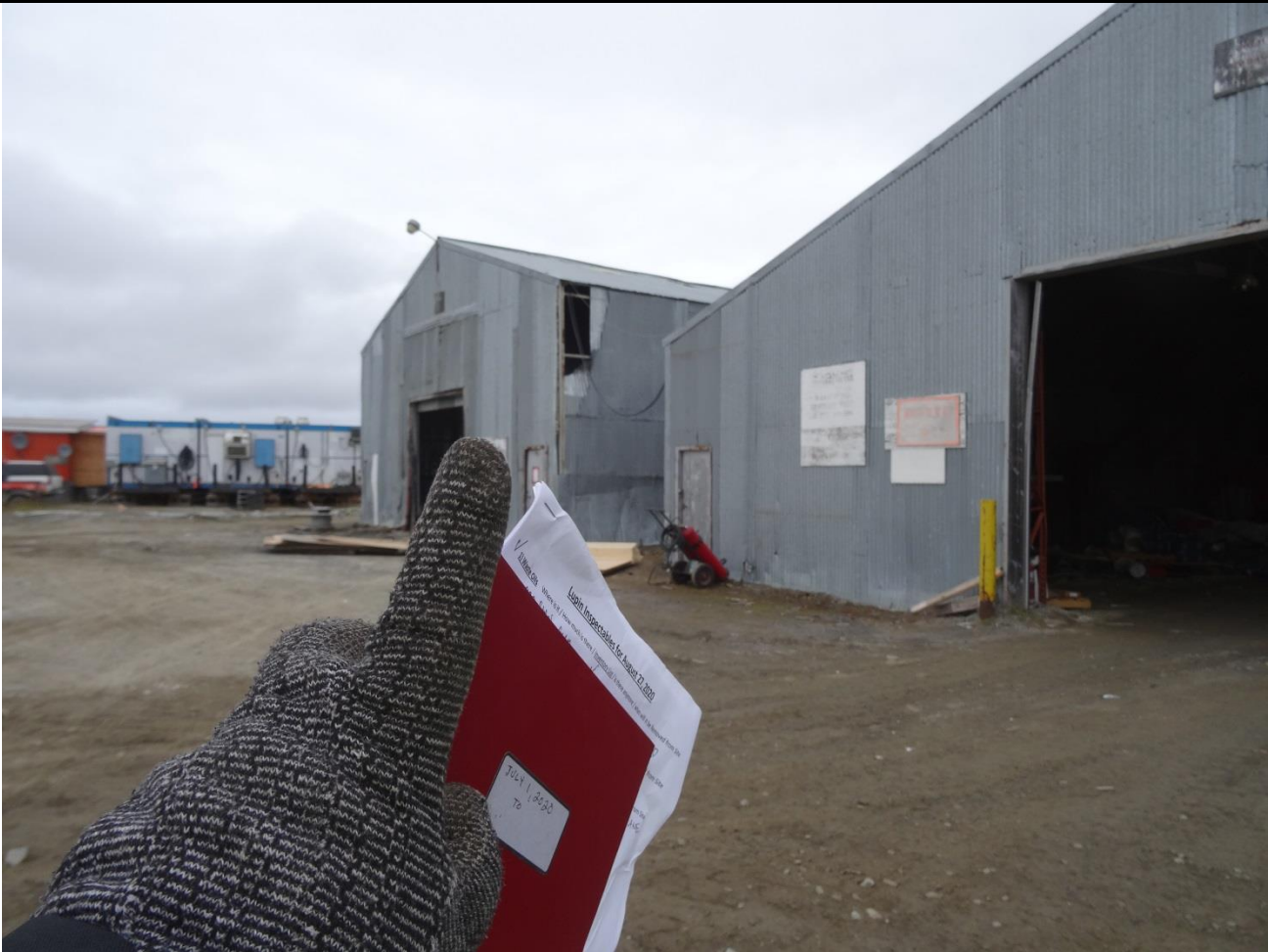
Description: Cold Storage Building #1 – On Left Side
