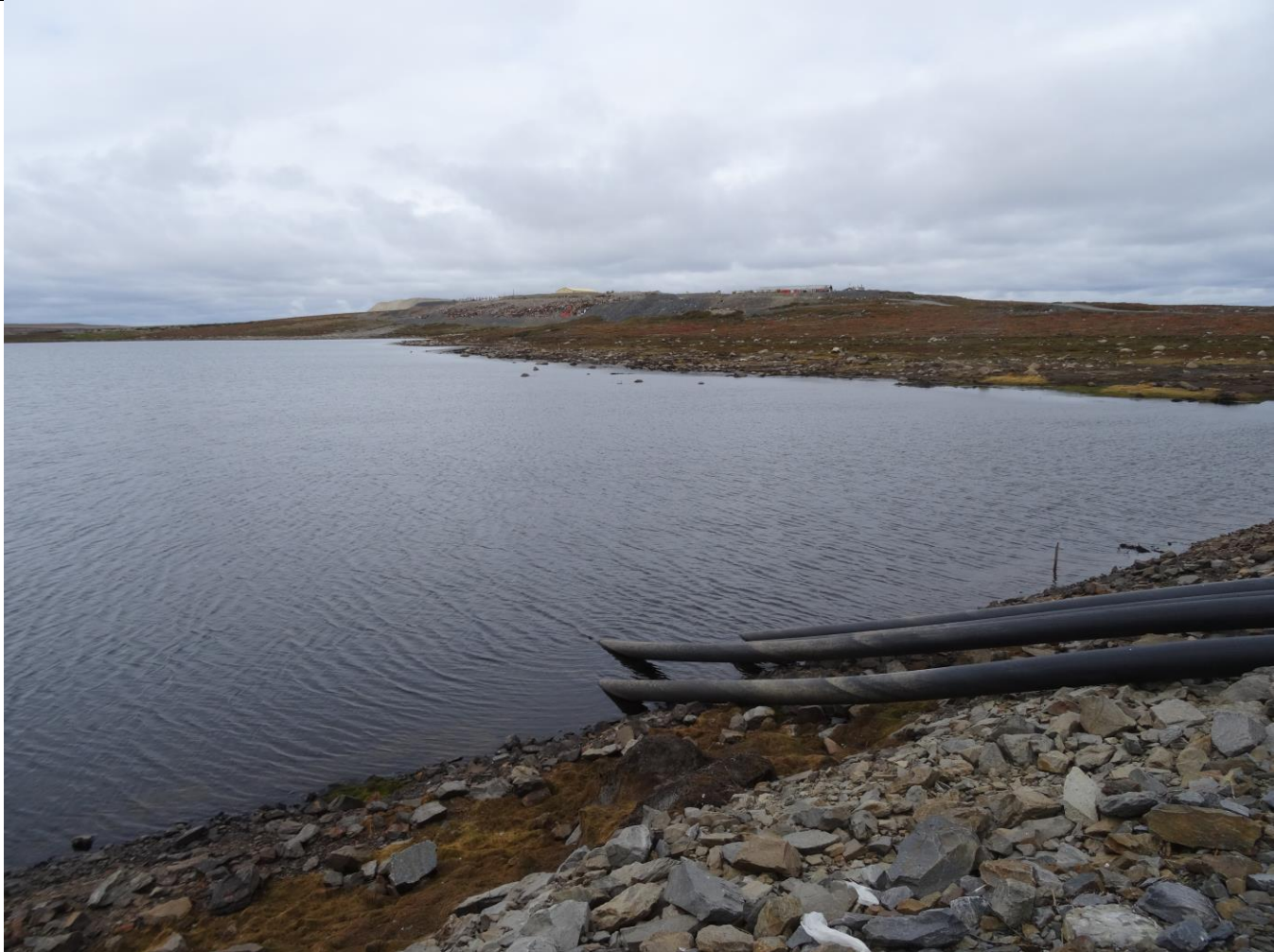
Description: Lower Sewage Lagoon
