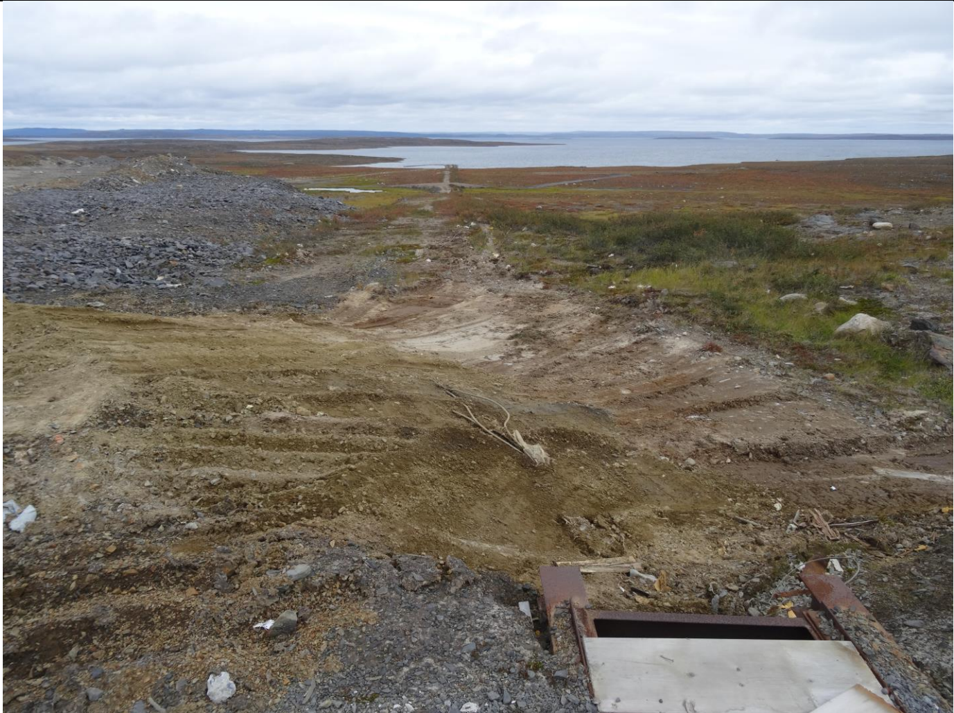
Description: Water Line – From here all the way down to Contwoyto Lake in the Background – ALL Debris Removed into the Land Fill
