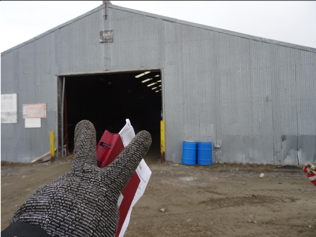
Description: Cold Storage Building #2, aka #20 ATV Building
