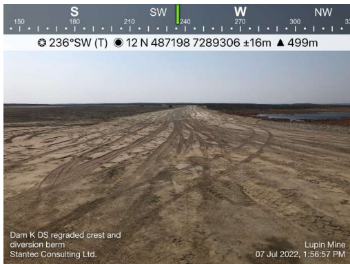
Photo 36: Looking southwest at the regraded crest and diversion berm of Dam K.
