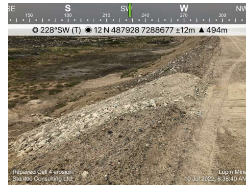
Photo 24: Looking southwest at the downstream crest of Dam 4 with the erosion repaired.
