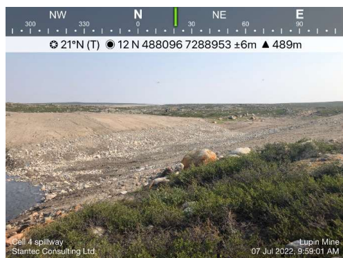
Photo 50: the newly constructed Cell 4 spillway through the Divider Dyke.
