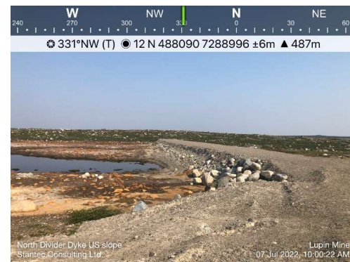
Photo 49: Looking northwest at the upstream slope of the north divider dyke.
