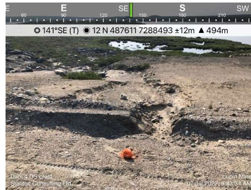
Photo 20: Looking southeast at the upstream slope of Dam 4 with erosion gully.
