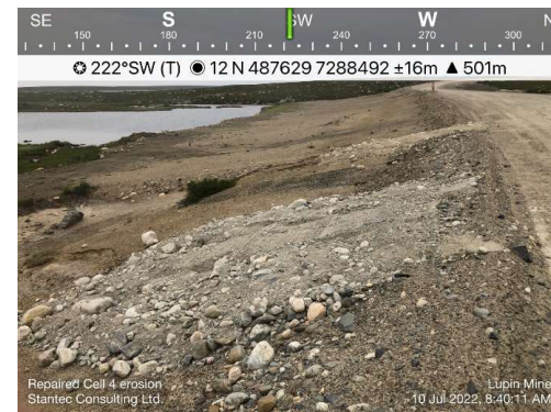
Photo 21: Looking southwest at the downstream crest of Dam 4 with the repaired completed over the erosion gully.
