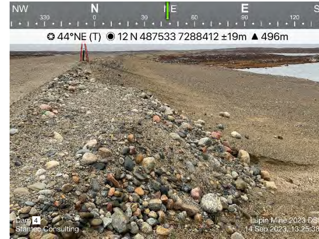
Photo 29: Overview of a previously repaired erosional feature on the downstream embankment at Dam 4.
