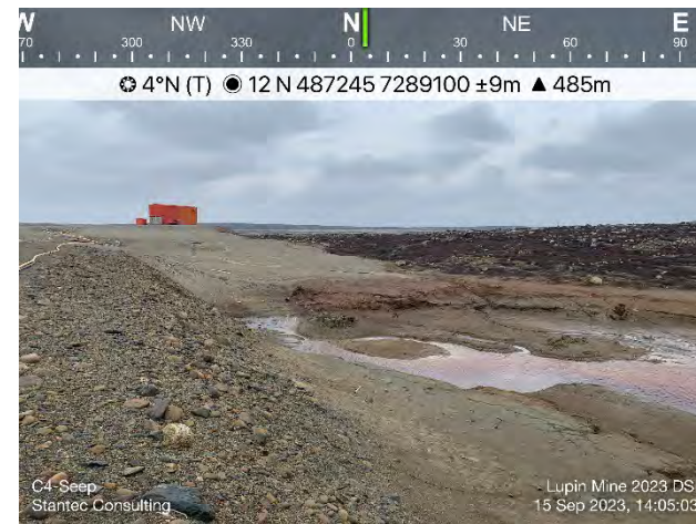
Photo 69: Overview of the NW corner of Cell 4 and the acidic seep.
