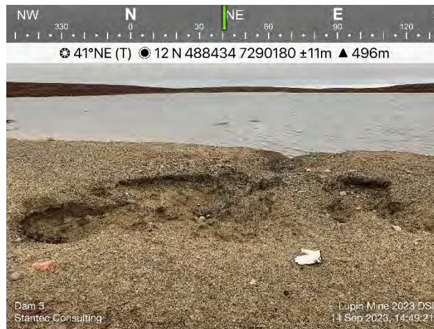
Photo 22: An erosional feature situated near the crest and on the downstream embankment of Dam 3.
