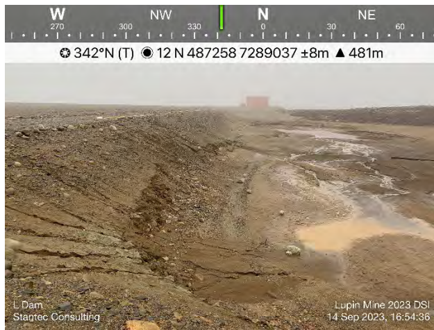
Photo 46: The downstream embankment and existing wave-action erosion at L Dam.
