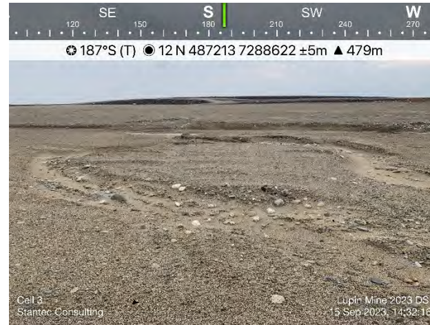
Photo 50: Overview of the Cell 3 drainage swale and localized erosional features adjacent to/within the swale.
