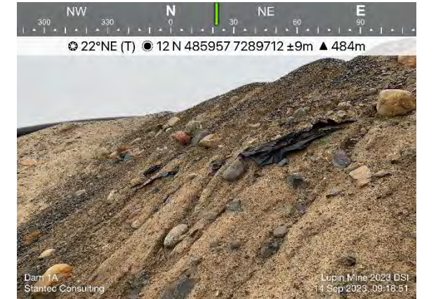
Photo 6: Exposed geotextile and existing, minor erosional features on the downstream embankment at Dam 1A.
