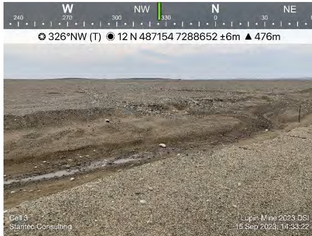
Photo 49: Overview of the Cell 3 drainage swale and localized erosional features adjacent to/within the swale.
