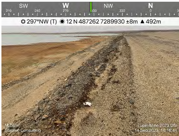
Photo 54: Existing tension cracking and erosion on the crest of M Dam.
