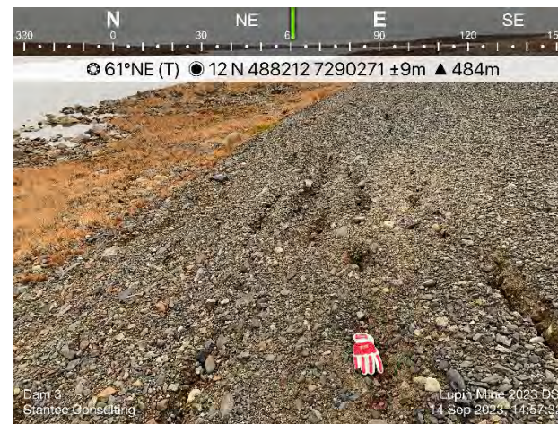
Photo 19: Tension cracking on the downstream embankment.
