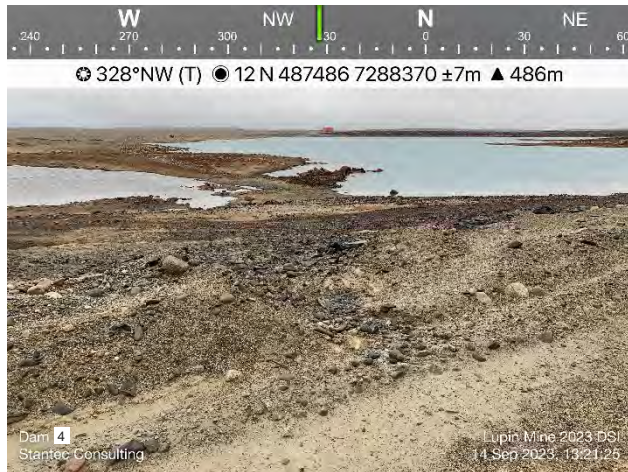
Photo 27: A small erosional feature located near the crest and on the upstream embankment of Dam 4.
