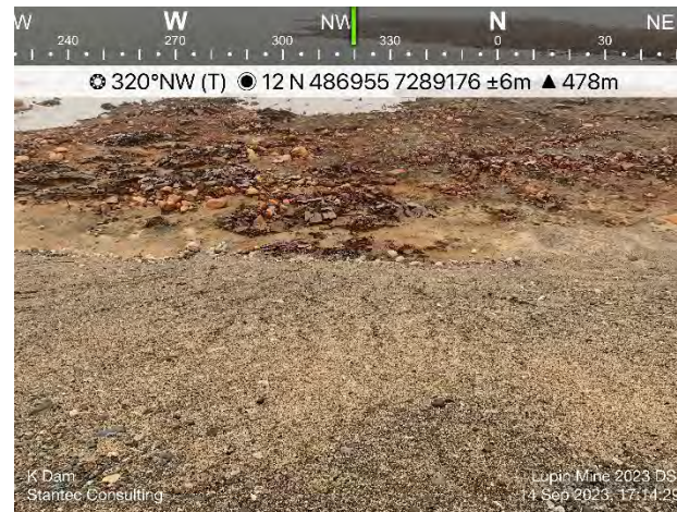
Photo 43: Rilling on the downstream embankment at K Dam.
