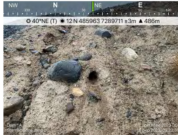
Photo 5: Close-up view of an animal burrow located approximately one metre below the crest. Minor erosional features (rills and small gullies) were also observed in the vicinity of this animal burrow.
