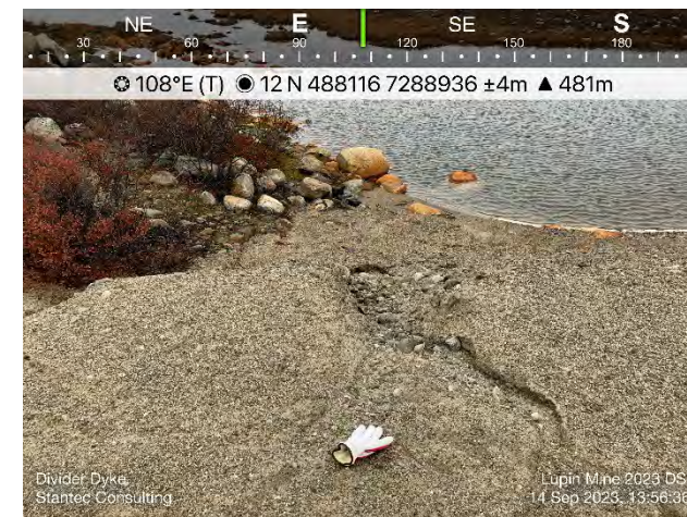
Photo 60: Existing erosional feature near the crest and on the embankment of the South Divider Dyke.
