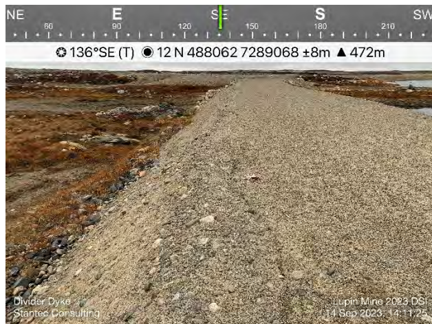
Photo 61: Existing tension crack on the crest near the downstream embankment on the South Divider Dyke.
