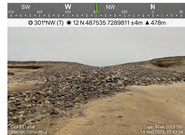
Photo 41: Overview of the Cell 5 outfall structure that was incorporated in J Dam in 2021.
