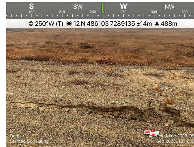
Photo 14: Instance of a small erosional feature extending from the crest to the downstream embankment at Dam 1C.
