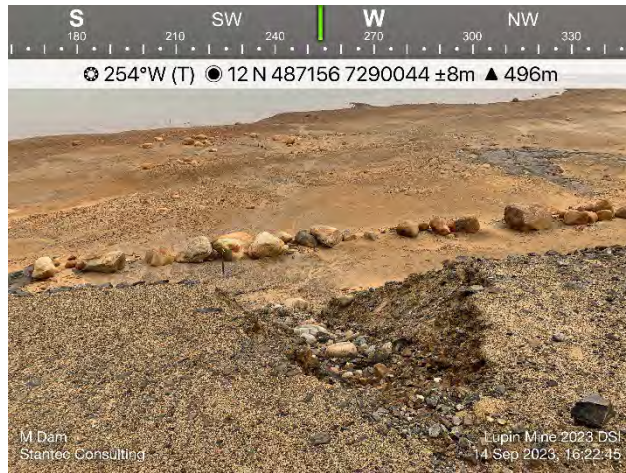
Photo 55: Fresh erosional feature on the crest and downstream embankment at M Dam.
