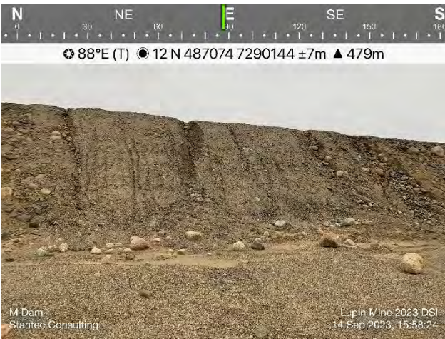
Photo 53: Fresh erosional features on the downstream embankment at M Dam.
