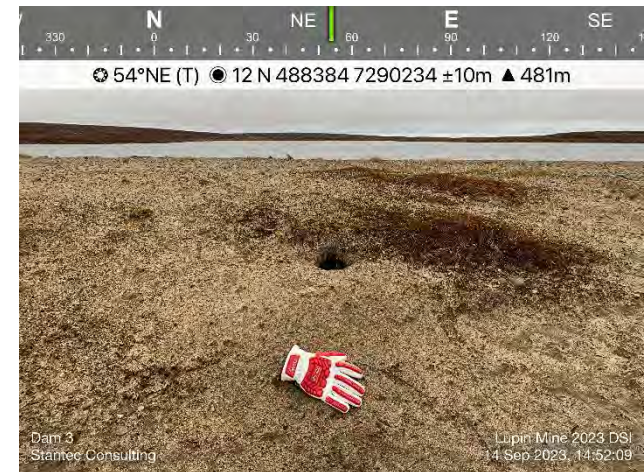
Photo 23: Animal burrow located near the crest of Dam 3.
