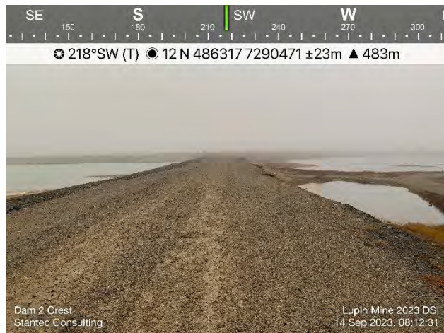
Photo 15: Overview of the crest and the north seepage collection pond at Dam 2. The seepage collection pond had water present at the time of inspection, presumably related to runoff and not seepage.
