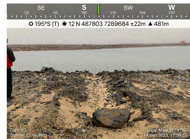
Photo 38: Existing erosional feature near the crest on the downstream embankment at Dam 3D.
