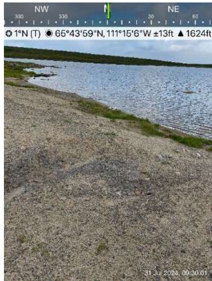
Photo 25: Erosional feature developing on the downstream embankment of Dam 3.
