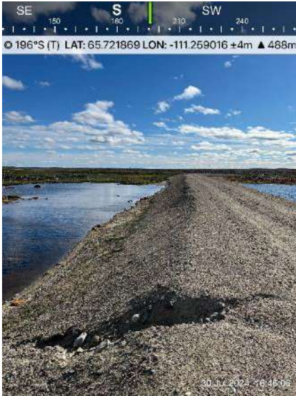
Photo 61: Existing erosional feature on the crest and downstream embankment on the South Divider Dyke.
