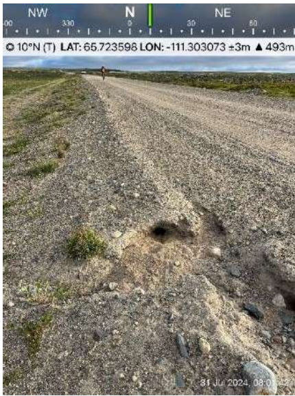
Photo 14: Instance of a small erosional feature extending from the crest to the downstream embankment at Dam 1C.
