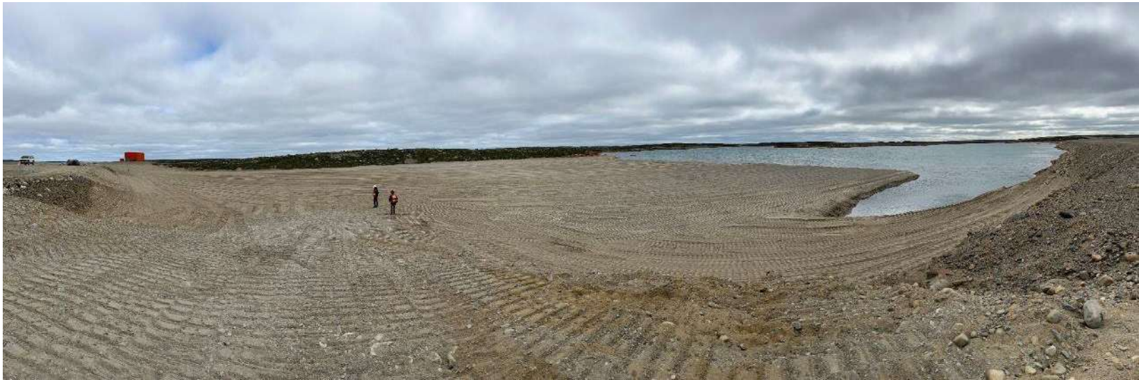
Photo 52: Overview of the esker cover placed over previously exposed tailings and the limestone drain in the NW corner of Cell 4.
