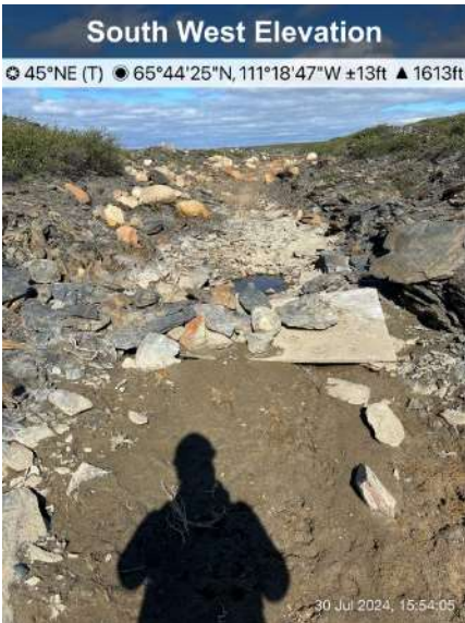
Photo 64: Plywood and small rock check dam in the Divider Dyke spillway.
