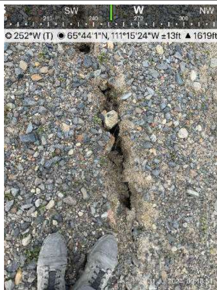
Photo 21: Close up of the tension cracking on the downstream embankment.
