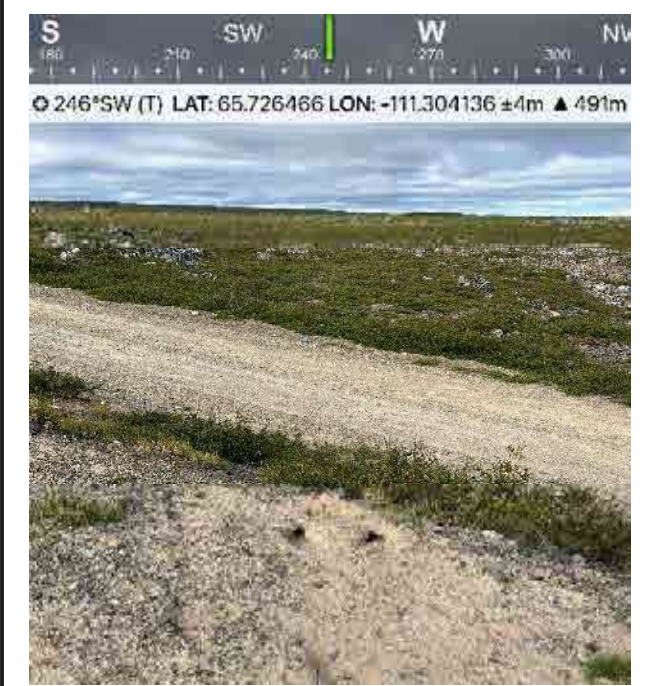
Photo 10: Two small animal burrows situated near the crest of Dam 1B.
