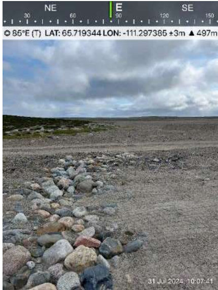
Photo 37: Overview of the surface water management feature on Dam 6.
