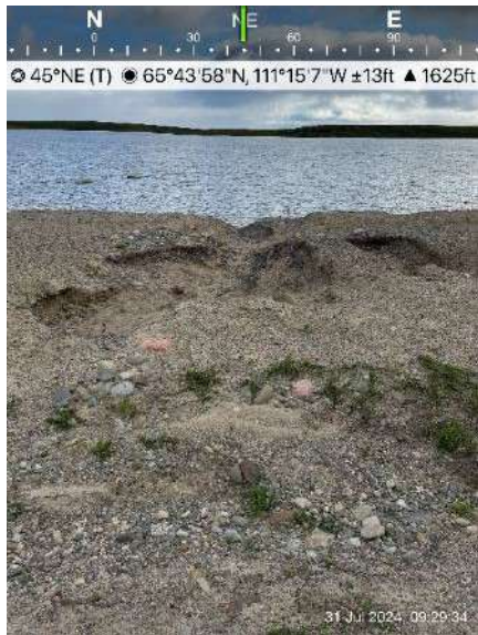
Photo 24: An erosional feature situated near the crest and on the downstream embankment of Dam 3.
