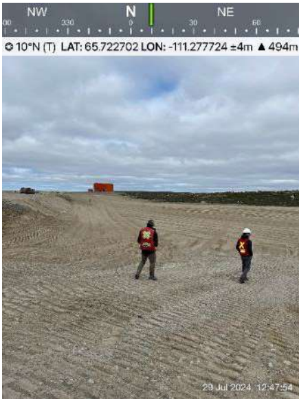
Photo 49: Esker cover placed over the installed limestone drain in the NW corner of Cell 4, looking north.
