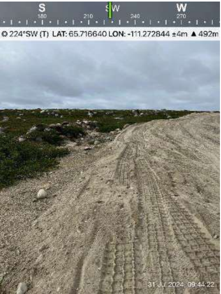
Photo 29: Dam 4 southwest abutment. The windrows were graded and tied into natural ground at the abutment.
