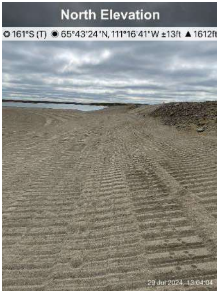
Photo 50: Esker cover placed over the limestone drain on Cell 4, looking south.
