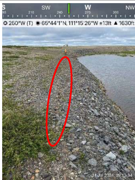
Photo 20: Tension cracking on the downstream embankment, circled in red.
