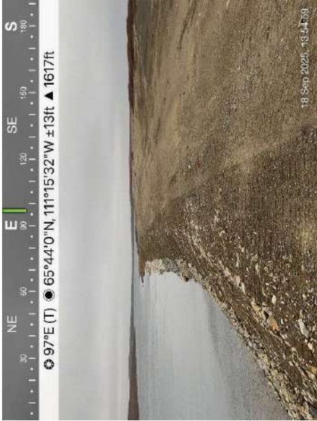
Photo 12: Overview of the Dam 3 crest and downstream embankment. Resloping work was completed in September, and riprap placed at the toe.
