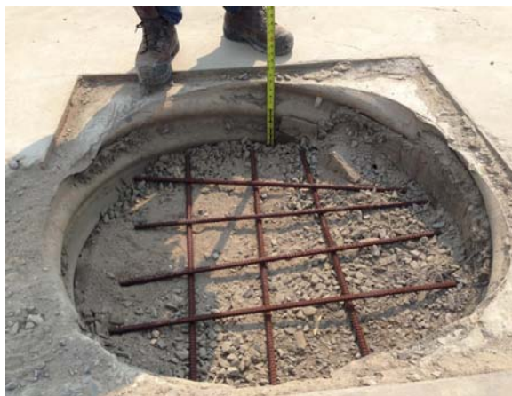
Photo 2: Rebar reinforcement within the drain outlet.
