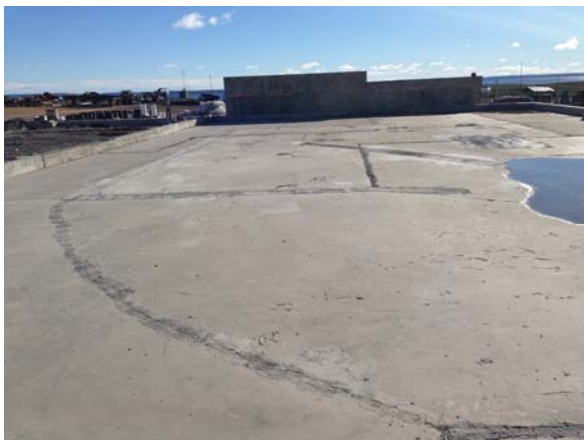
Photo 7: Grouting the cracks on the foundation pad.
