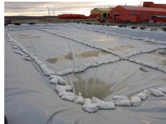
Photo 12: Deployed liner with sand bags and old tires as ballast.
