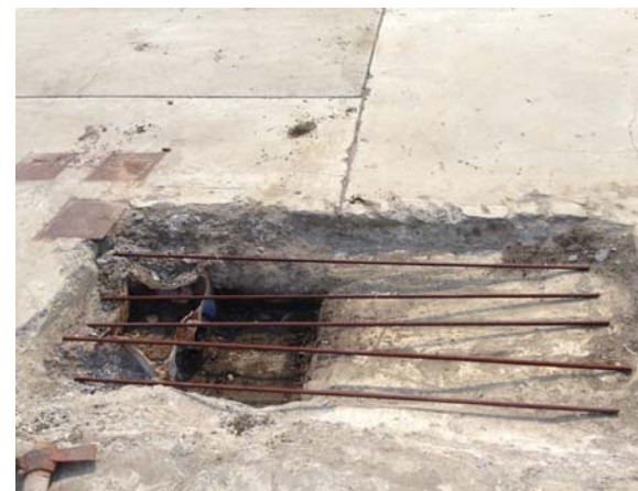
Photo 3: Rebar reinforcement within the drain outlet.
