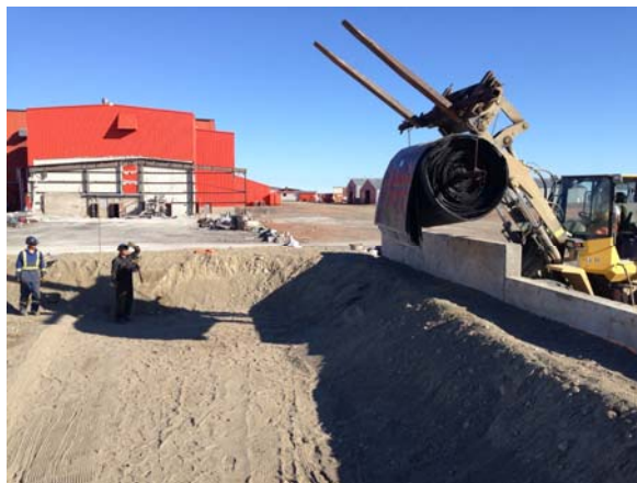
Photo 8: Liner deployment over the finished subgrade.
