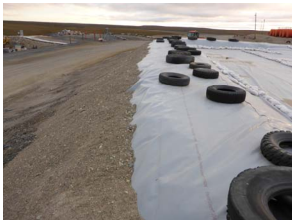
Photo 16: Liner edge are buried within the exterior slope.
