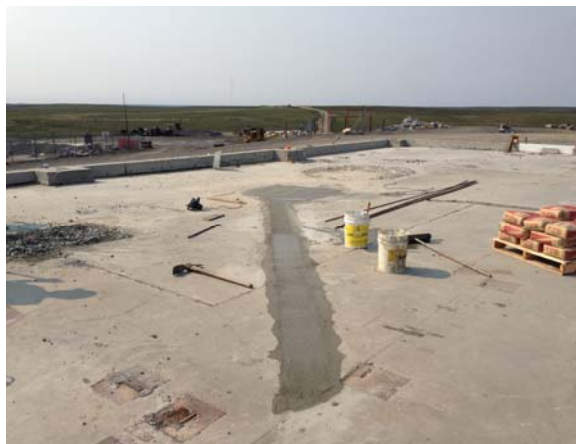
Photo 5: concrete backfill in the channel and outlets.
