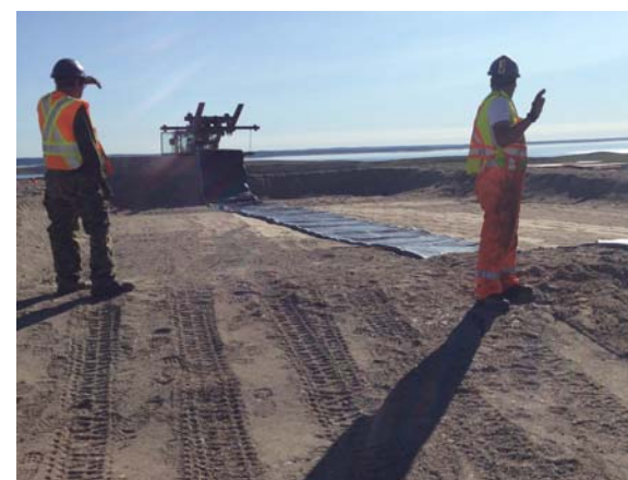
Photo 9: Liner deployment continued.
