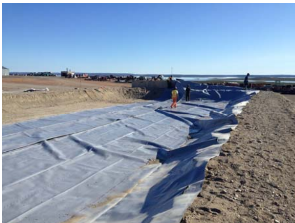
Photo 10: Liner deployment continued.
