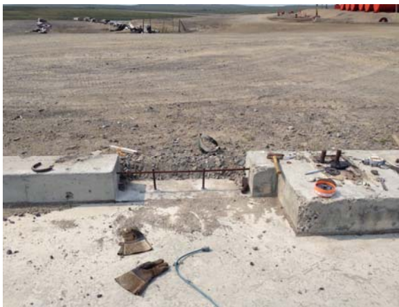
Photo 4: Rebar reinforcement between an old doorway.
