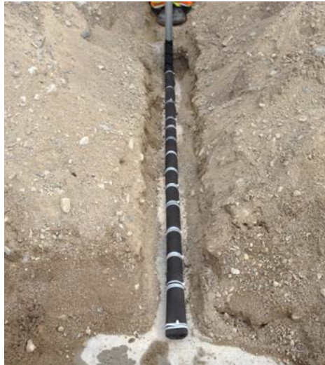
Photo 13: Horizontal section of the leakage detection pipe wrapped with geotextile within the subgrade.
