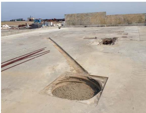
Photo 1: Clearing of the concrete foundation and removal of debris in drain outlets
