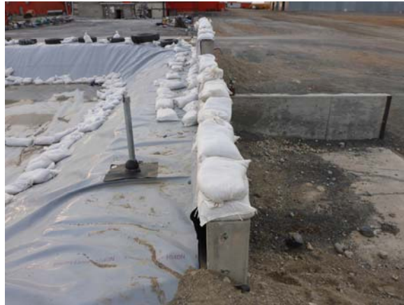
Photo 14: View of the leakage detection pipe at the east end of the landfarm, between the sump and the raised concrete footing.
