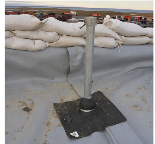
Photo 15: Close up view of the sampling port of the leakage detection pipe.
