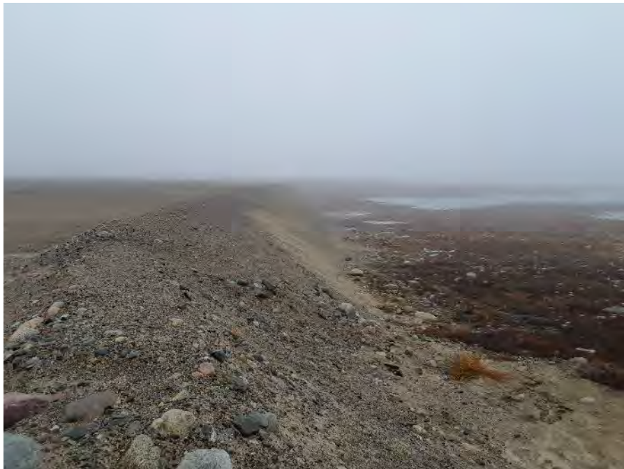
Photo 44: K Dam downstream slope, recently regraded, facing southwest (Fig. A1 ID#91)
