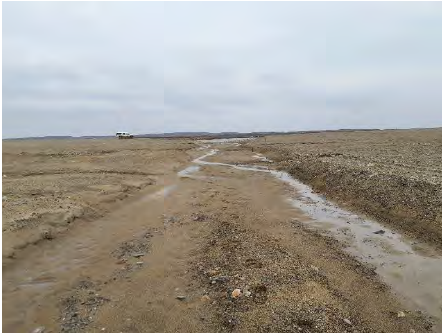
Photo 52: M Dam erosion rills on downstream slope, facing northeast (Fig. A1 ID#71)
