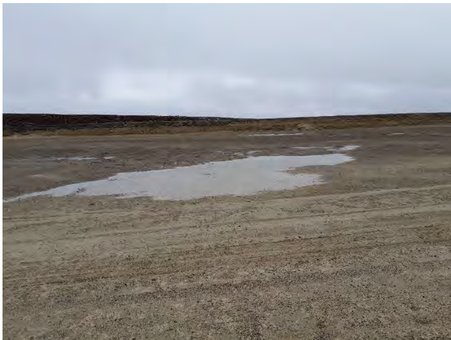
Photo 64: N Dam ponded water on cover upstream of dam, facing east (Fig. A1 ID#67)
