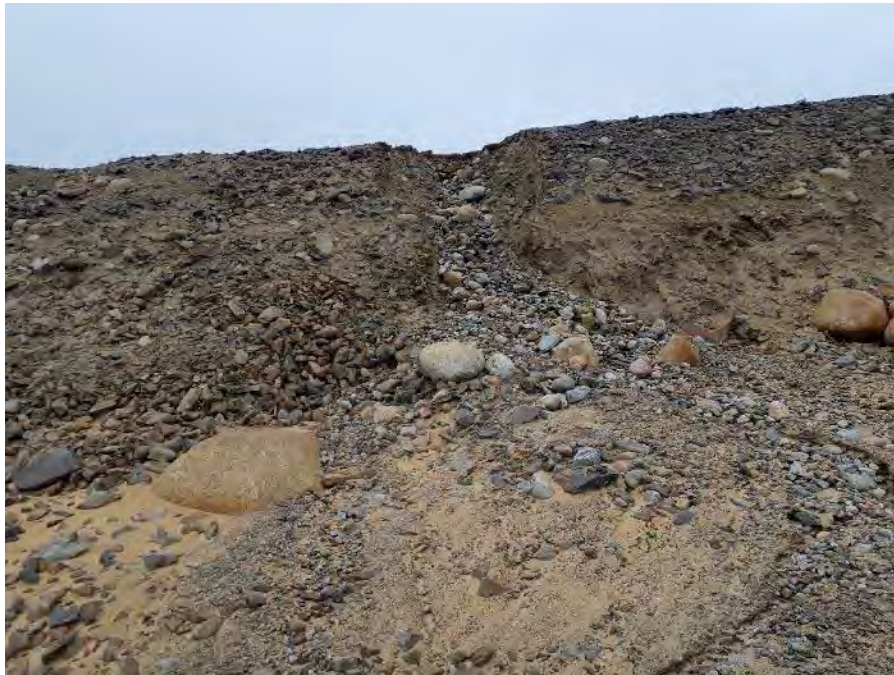
Photo 54: M Dam erosion rill facing southwest from crest, exposed tailings in background (Fig. A1 ID#79)
