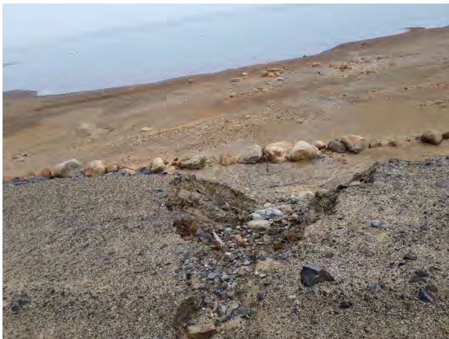
Photo 54: M Dam erosion rill facing southwest from crest, exposed tailings in background (Fig. A1 ID#79)
