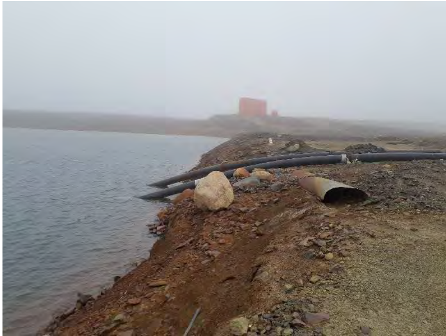
Photo 42: J Dam, four 0.2m diameter pipes throughgoing the dam for overflow control, appear undersized (Fig. A1 ID#83)
