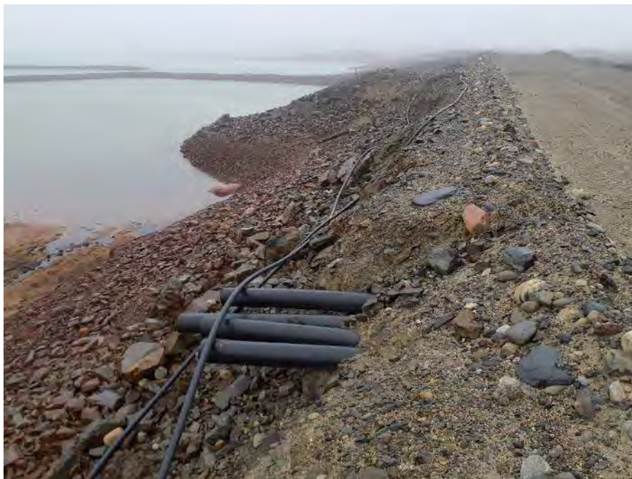
Photo 42: J Dam, four 0.2m diameter pipes throughgoing the dam for overflow control, appear undersized (Fig. A1 ID#83)
