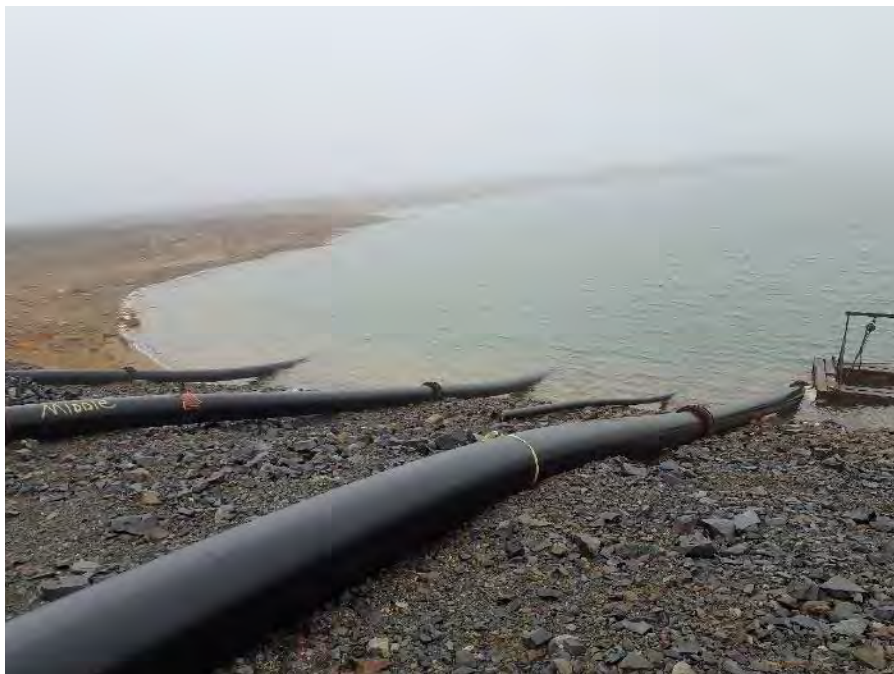
Photo 6: Dam 1A syphon pipes in Pond 2 (Fig. A1 ID#22)
