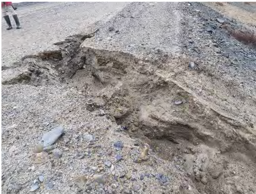
Photo 28: Dam 4 erosion rill in crest and downstream slope, facing east (Fig. A1 ID#49)
