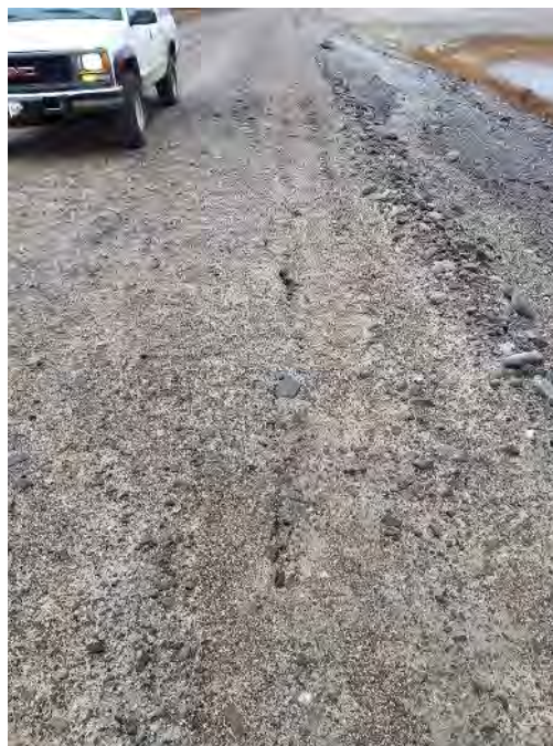
Photo 34: Dam 6 longitudinal cracks near upstream shoulder of crest, facing northwest (Fig. A1 ID#35)
