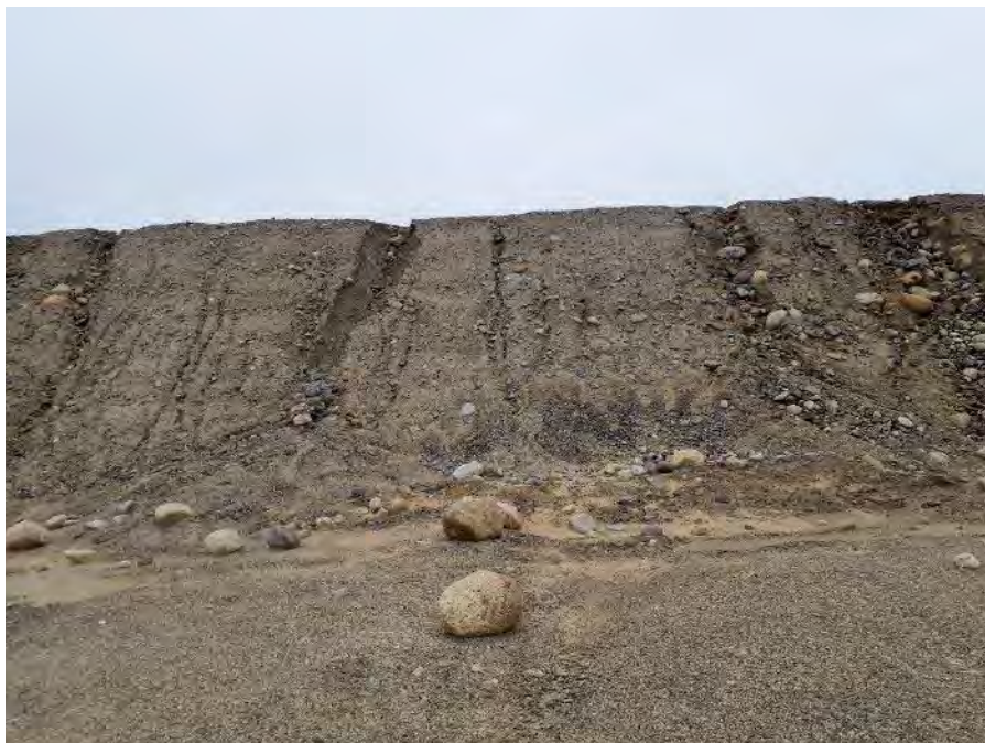
Photo 52: M Dam erosion rills on downstream slope, facing northeast (Fig. A1 ID#71)
