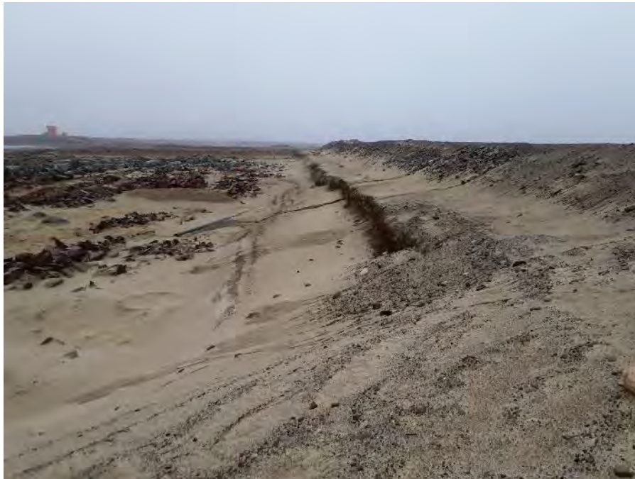
Photo 44: K Dam downstream slope, recently regraded, facing southwest (Fig. A1 ID#91)
