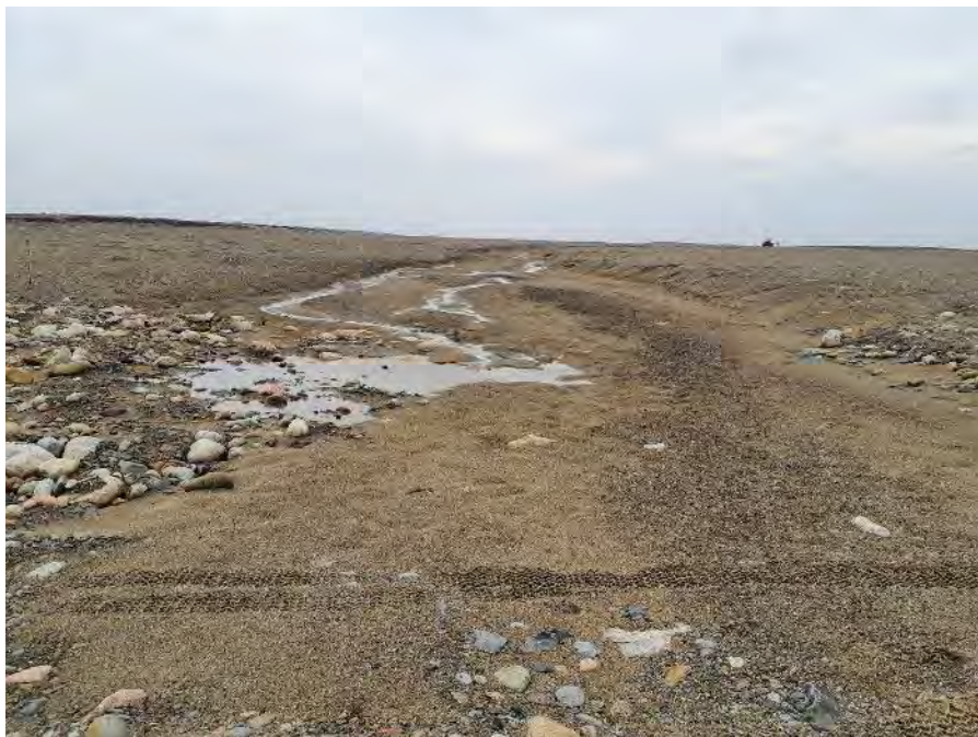
Photo 50: Cell 3 outfall structure erosion on channel slopes (Fig. A1 ID#107)
