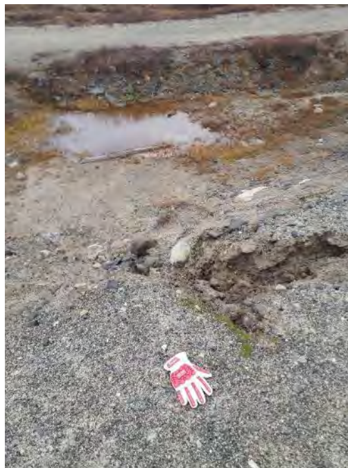
Photo 14: Dam 2 erosion rill on downstream slope (Fig. A1 ID#2)
