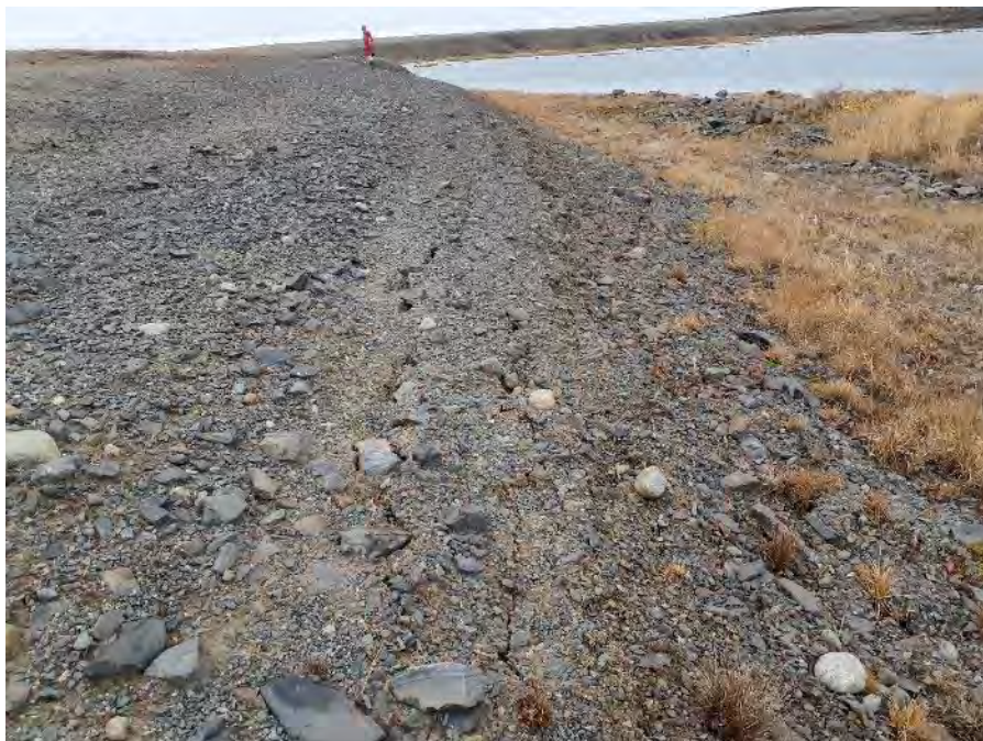
Photo 22: Dam 3 longitudinal cracks near downstream toe, facing west (Fig. A1 ID#61)
