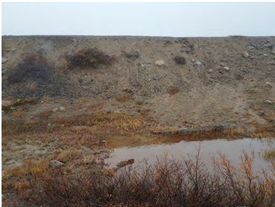
Photo 16: Dam 2 downstream slope sloughing (Fig. A1 ID#9)
