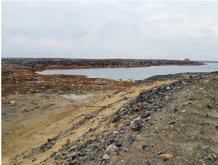
Photo 40: Dam 3D downstream slope, high water mark evident at toe (Fig. A1 ID#112)
