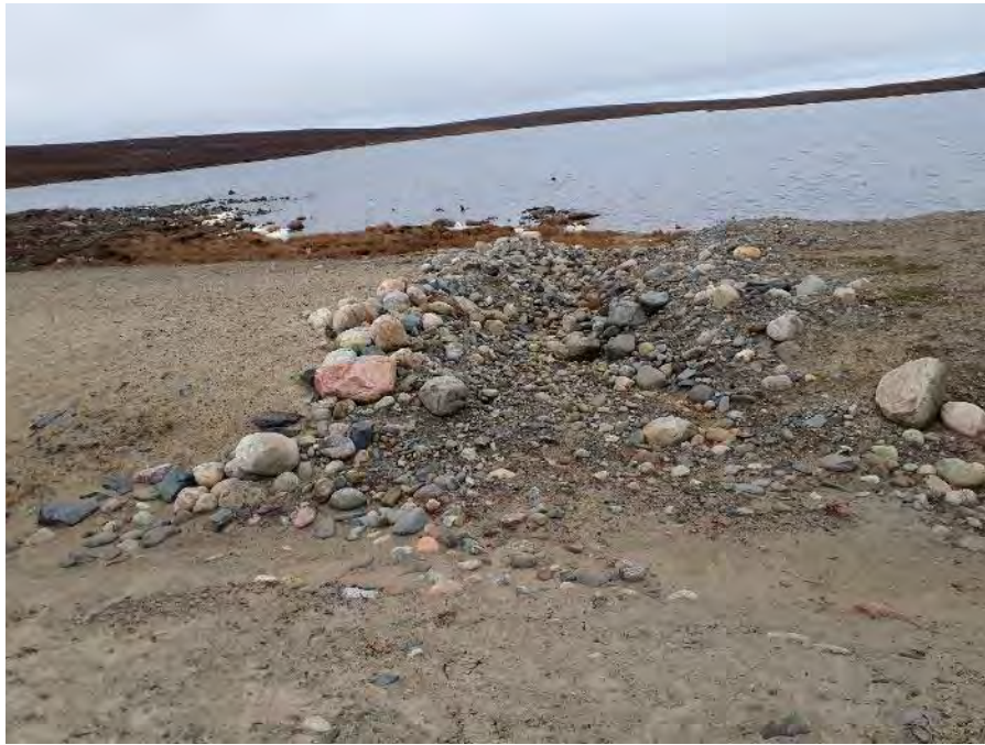
Photo 20: Dam 3 drainage channel in downstream slope, facing north (Fig. A1 ID#60)
