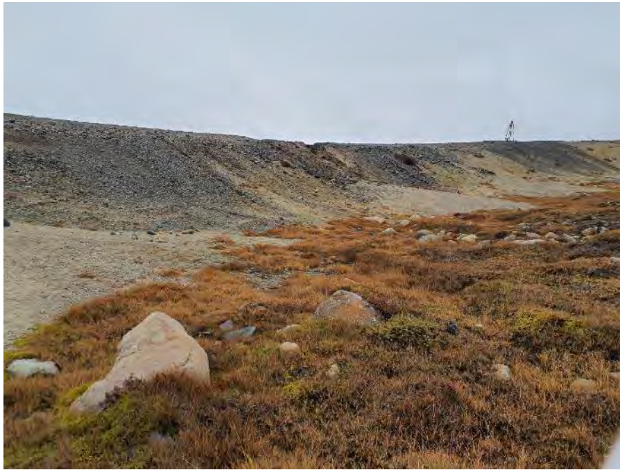
Photo 28: Dam 4 erosion rill in crest and downstream slope, facing east (Fig. A1 ID#49)
