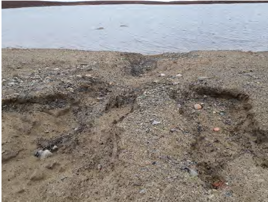
Photo 22: Dam 3 longitudinal cracks near downstream toe, facing west (Fig. A1 ID#61)
