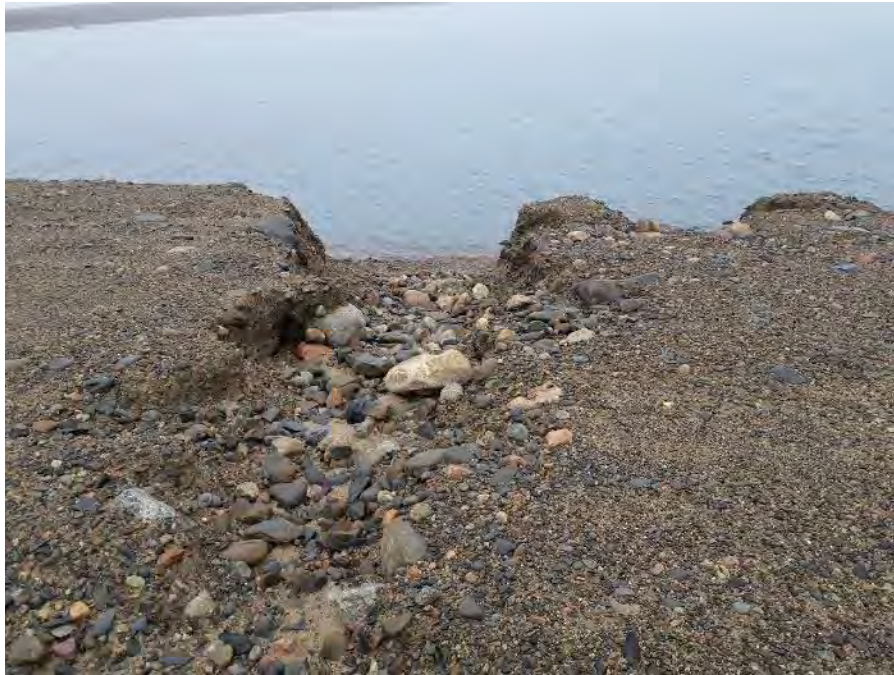
Photo 48: L Dam exposed tailings downstream of dam, facing north (Fig. A1 ID#87)
