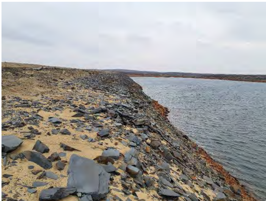
Photo 40: Dam 3D downstream slope, high water mark evident at toe (Fig. A1 ID#112)
