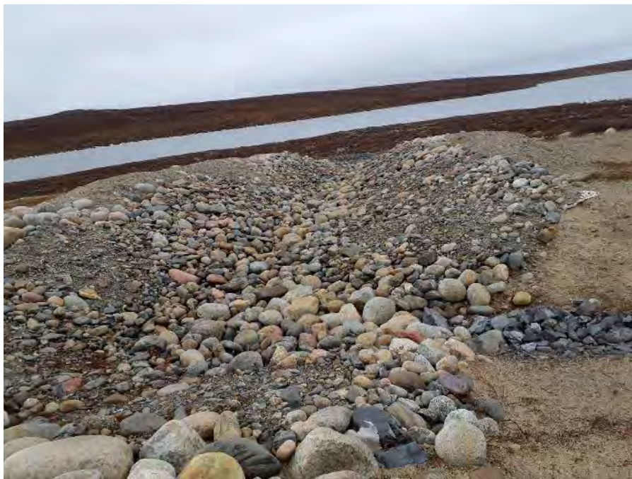
Photo 20: Dam 3 drainage channel in downstream slope, facing north (Fig. A1 ID#60)
