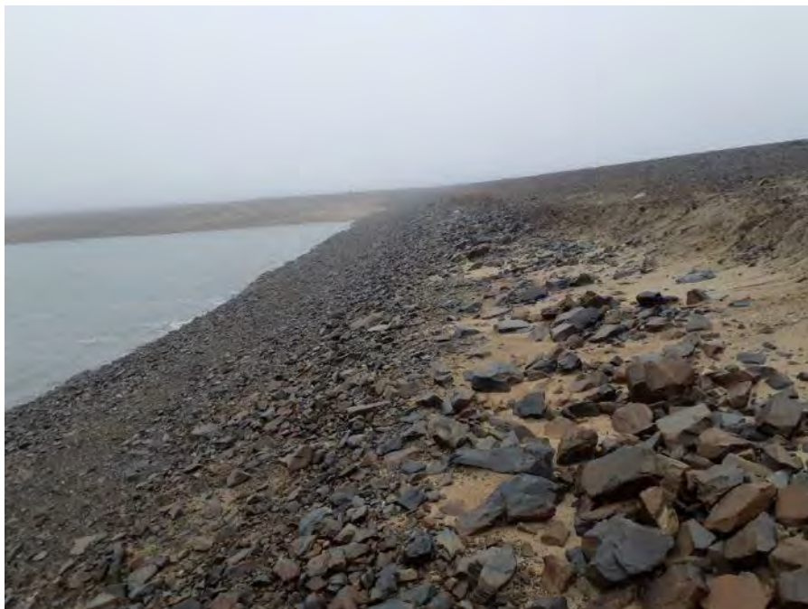
Photo 12: Dam 2 upstream slope riprap (Fig. A1 ID#4)
