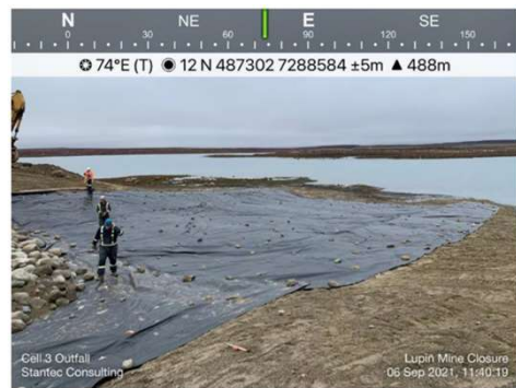
Photo 4: Geotextile fabric in Cell 3 outflow channel.
