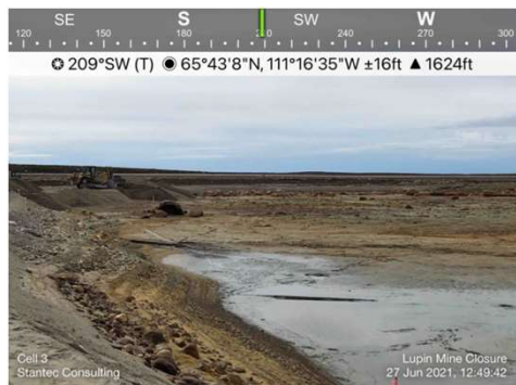
Photo 1: Esker cover placement in Cell 3. The cell has been dewatered prior to cover placement.
