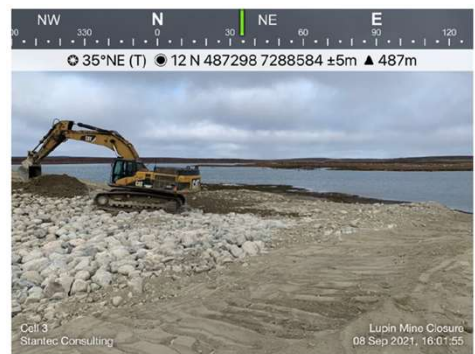
Photo 5: Excavator works to lay coarse material onto geotextile fabric in Cell 3 outflow channel.
