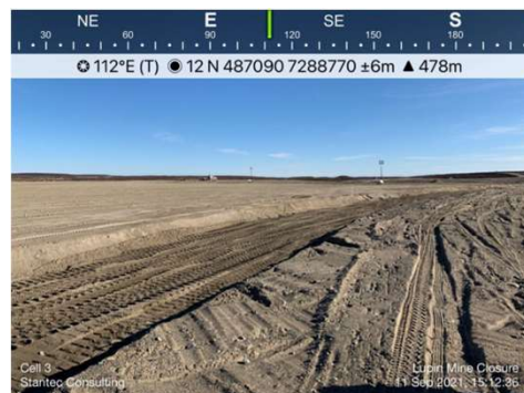
Photo 3: Completed Cell 3 esker cover. The cover surface was graded to be smooth and free draining.
