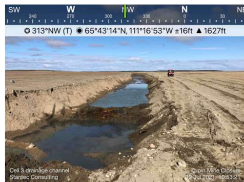
Photo 2: Cell 3 outflow channel during construction.
