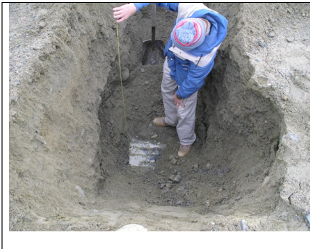
Photo 14. Test pit 1-1 in Cell 1, located at new pipe 7 installation
