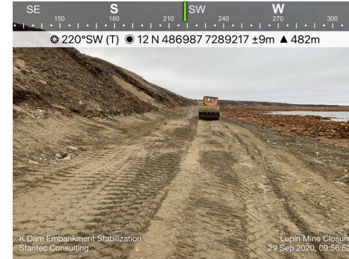
Photo 34: Looking southwest toward the south abutment of the reinforcement buttress with compaction being carried out
