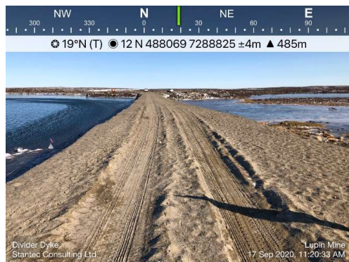
Photo 53: Looking north at the eroded crest slopes and sloughed crest of northern divider dyke.
