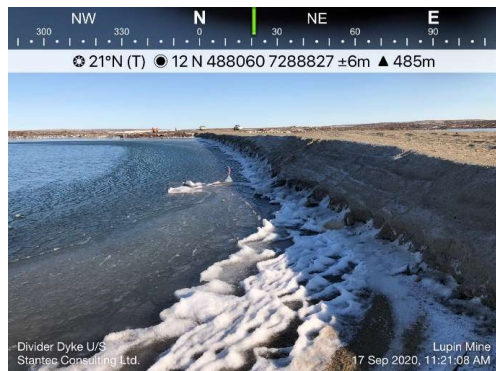
Photo 50: Looking north at the repaired upstream slope and crest of the southern divider dyke.
