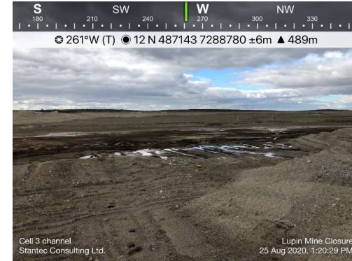
Photo 40: Looking west from Cell 3 onto the partially placed cover on exposed tailings.
