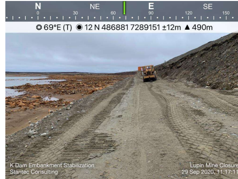
Photo 33: Looking east on the reinforcement buttress with compaction being carried out
