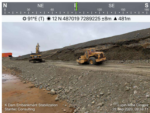
Photo 35: Looking east at the reinforcement buttress being constructed eroded toe at Dam K.
