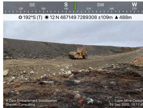
Photo 36: Looking south on the reinforcement buttress with compaction being carried out
